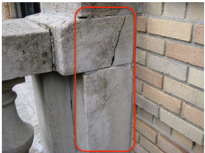
Fig. 2.29: Cracking in Portico Railing
