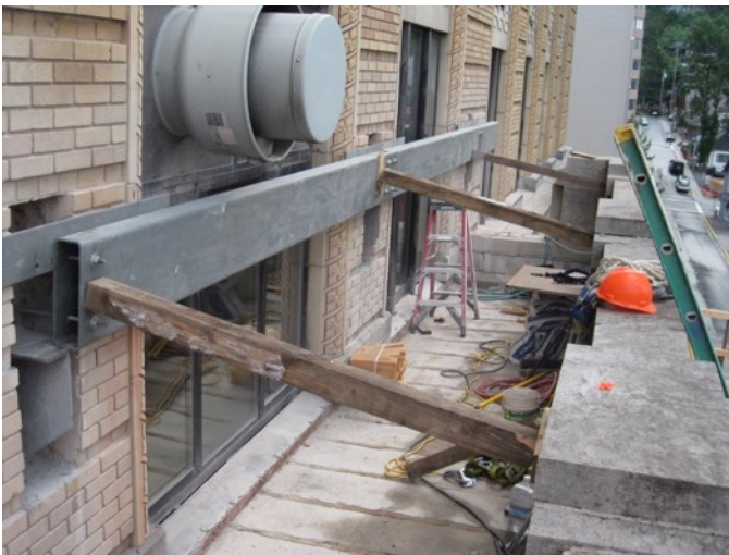
Fig. 5.3: Bracing of Building Masonry Fig. 5.4: Demolition of Portico Structure
