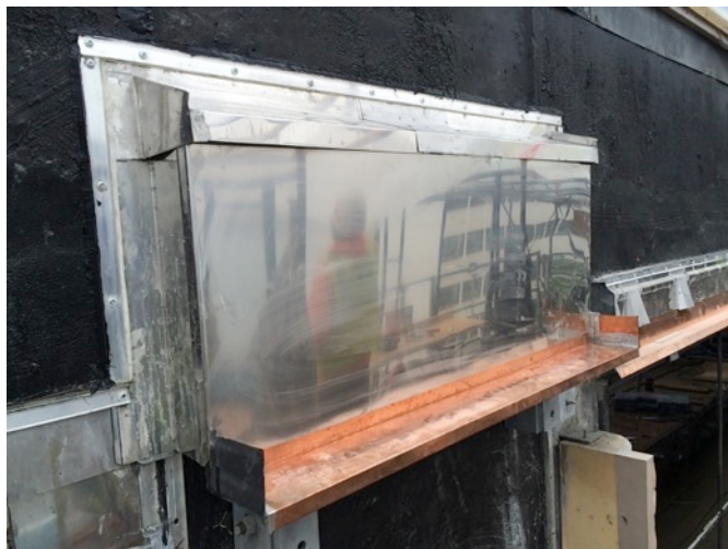
Fig. 5.54: Copper & St. Steel Ledger Flash'gs.
