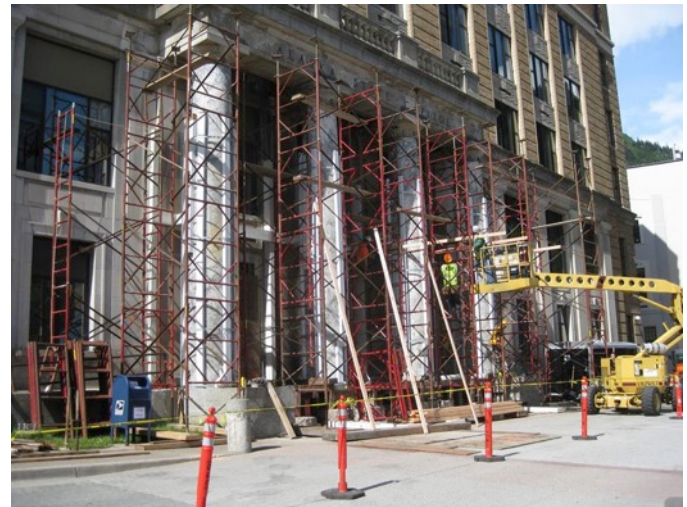
Fig. 5.1: Stairs Removed to Expose Found. Fig. 5.2: Bracing the Marble Columns
