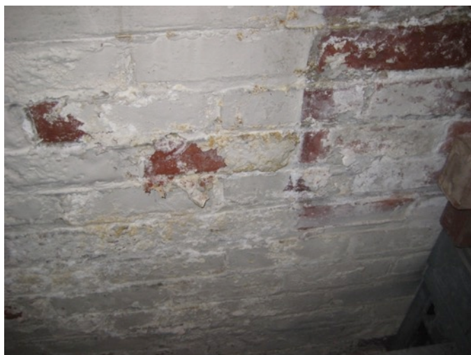
Fig. 3.95: Spalling Interior Brick Face
