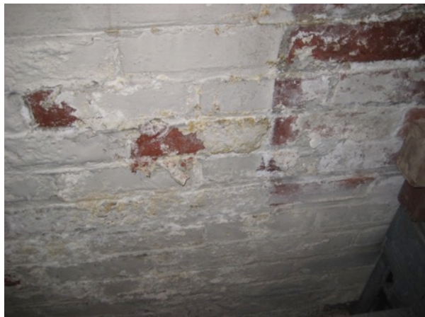
Fig. 3.57: Spalling & Efflor. on Int. Face Fig. 3.58: Spalling & Efflor. on Interior Face
