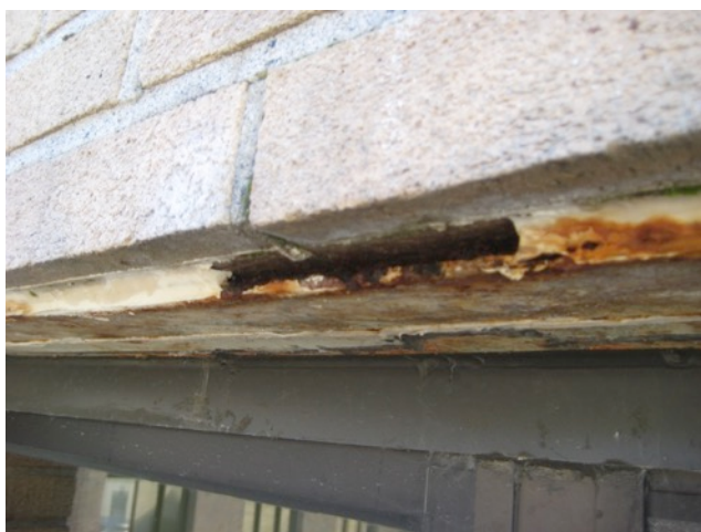
Fig. 3.68: Lintel Corrosion
