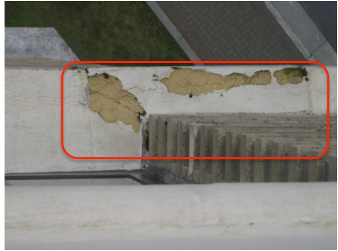
Fig. 3.18: Spalling Level 5 Terra-Cotta Band
