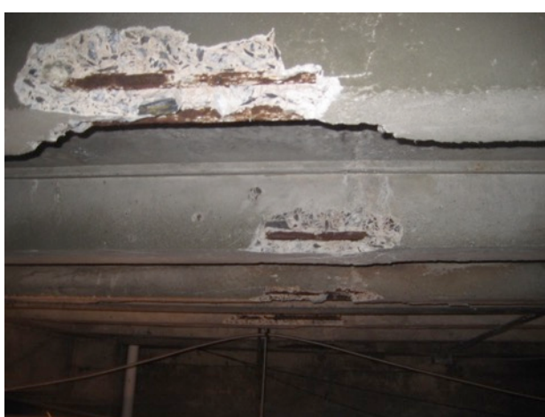
Fig. 3.86: Corrosive Spalling of Fl. Joist
