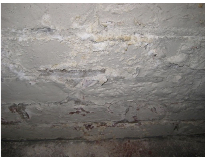
Fig. 3.96: Spalling Interior Brick Face
