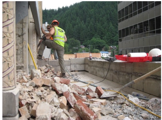
Fig. 5.3: Bracing of Building Masonry Fig. 5.4: Demolition of Portico Structure
