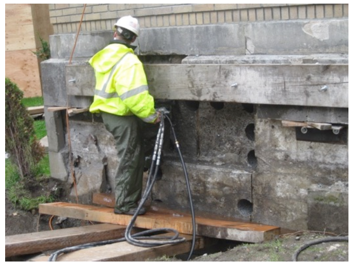
Fig. 5.29: Cutting Crawspace Access Hole
