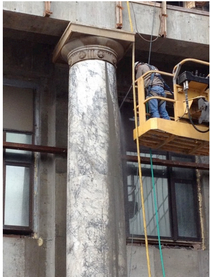
Fig. 5.25: Grouting Column Reinforcing
