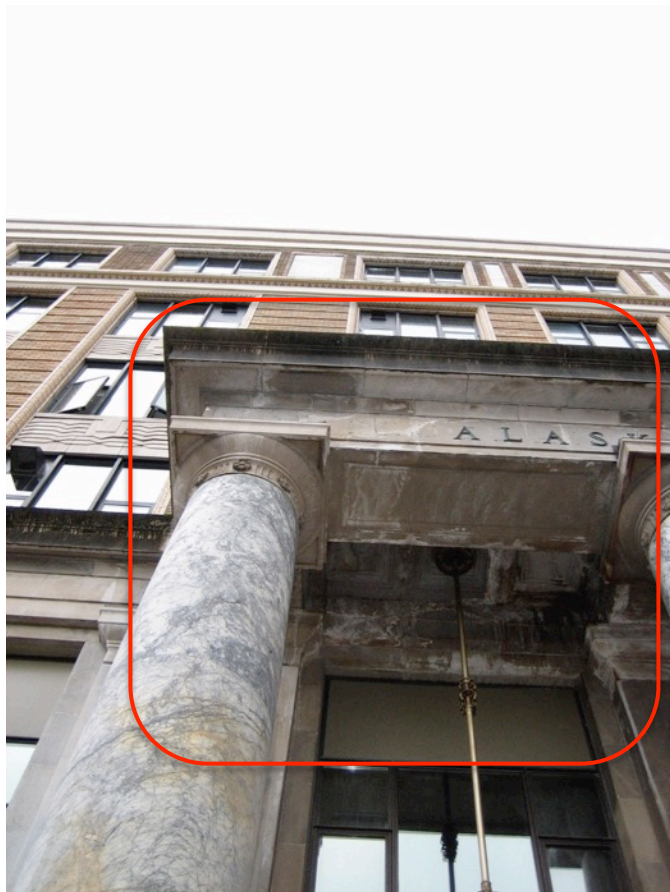
Fig. 2.33: Severe Staining of Portico Ceiling
