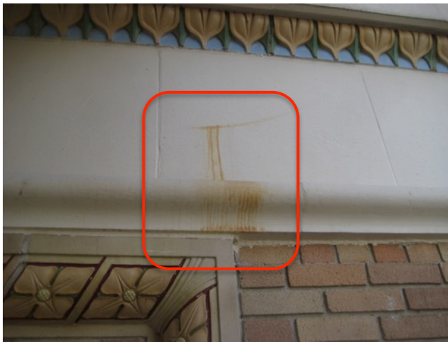
Fig. 3.19: Oozing Oxide Stain @ Lev. 5 T.-C.
