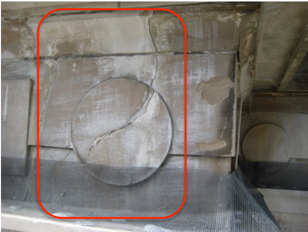
Fig. 2.7: Cracked Stone Beam End
