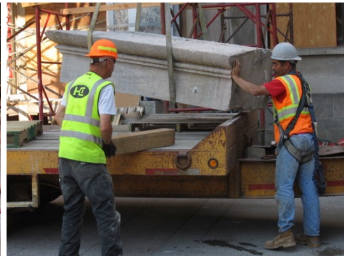
Fig. 5.8: Removal of Portico Beam
