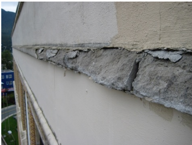
Fig. 3.1: Spalling Roof-Level Band
