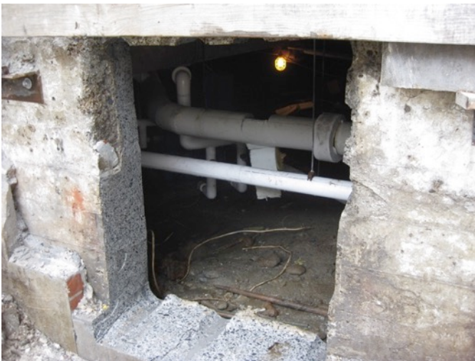
Fig. 5.30: Crawspace Access Hole
