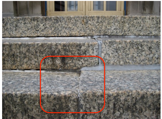
Fig. 2.26: Downward Displacement at Stair
