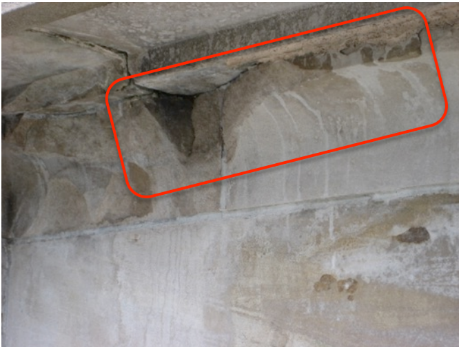
Fig. 2.3: Spalled-Off Chunk of Stone
