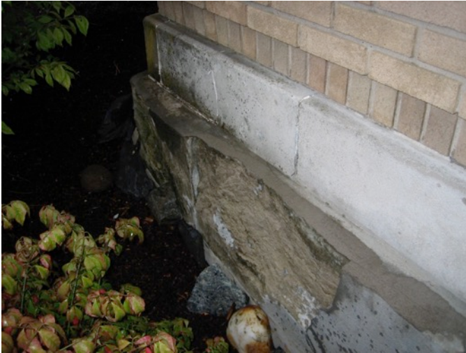
Fig. 1.1: Degradation of Stone Base
