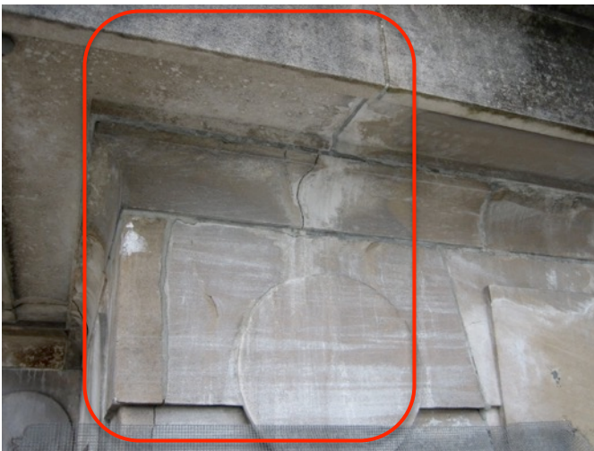
Fig. 1.15: Cracking of Stone Portico Beams
