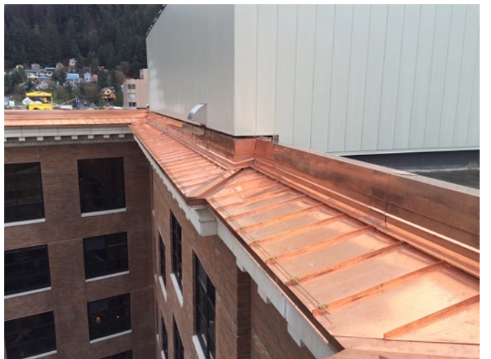
Fig. 5.81: Copper Roof Atop Cornice
