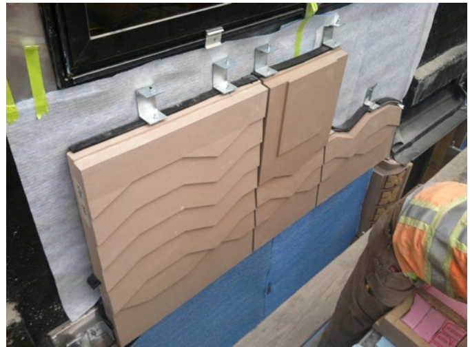
Fig. 5.68: Start of T.-C. Spandrel Installation Fig. 5.69: Terra-Cotta Spandrel Installation
