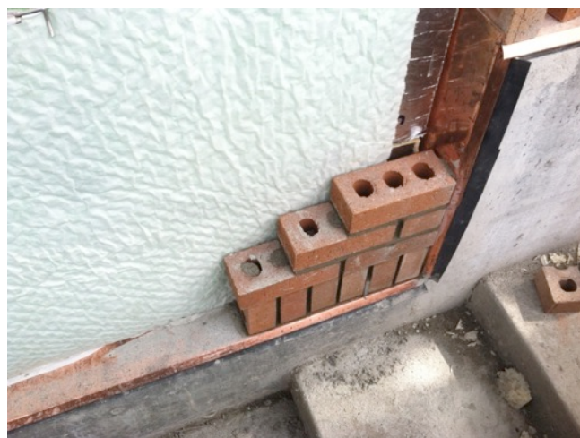
Fig. 5.46: Brick Veneer Resembles Existing
