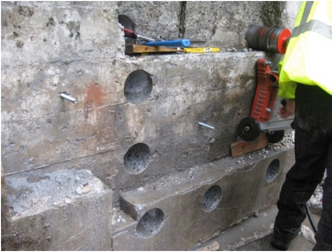
Fig. 5.28: Cutting Crawspace Access Hole
