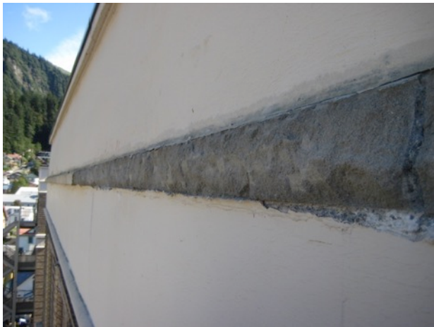
Fig. 3.3: Spalling Roof-Level Band
