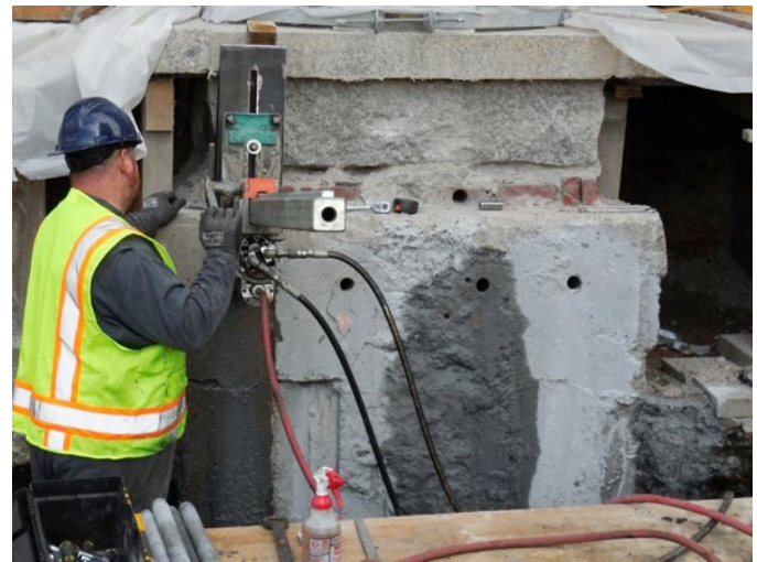
Fig. 5.15: Retrofitting Foundation Reinf.
