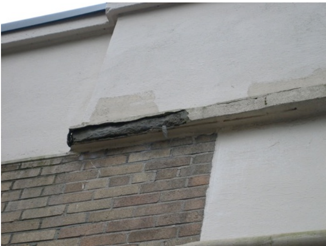
Fig. 1.9: Spalling Stone Cornice Band
