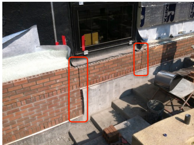
Fig. 5.50: Brick Exp. Joints @ Stress Lines
