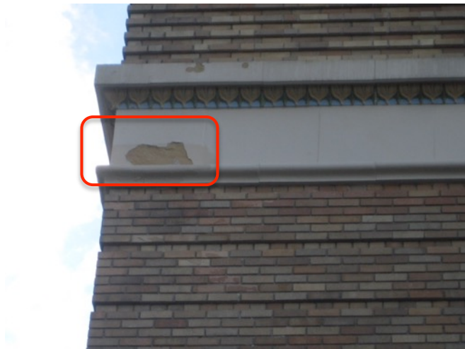
Fig. 3.11: Spalling Level 5 T.-C. Band
