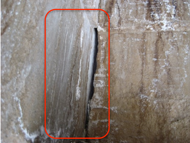
Fig. 2.1: Separation of Stone Beams
