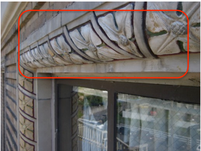
Fig. 3.27: Lime-Stained Window Surround
