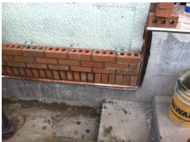
Fig. 5.47: New Brick Veneer Cladding
