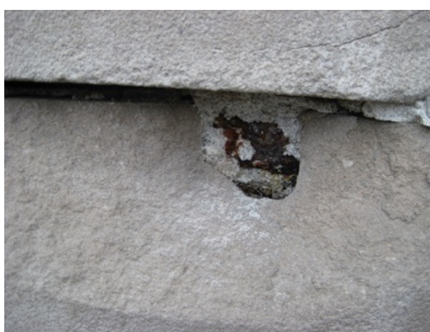
Fig. 3.46: Spall Due to Anchor Corrosion
