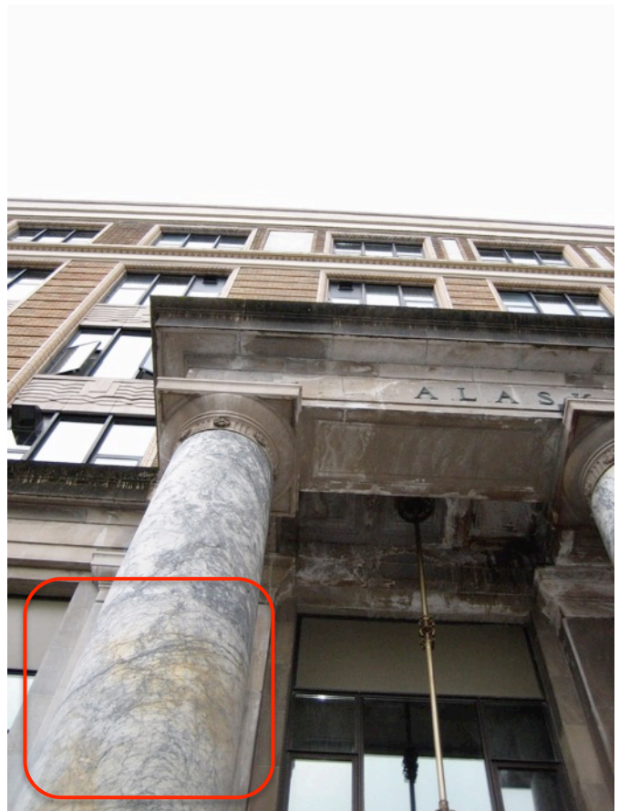
Fig. 2.14: Oxide Staining on Portico Column
