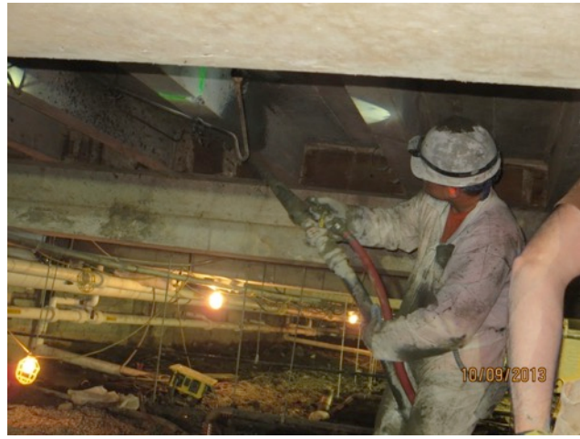
Fig. 5.35: Shot-Creting Damaged Joist
