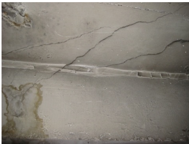
Fig. 3.82: Cracking of Floor Slab
