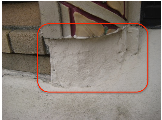
Fig. 3.26: Spalled T.-C. Window Surround
