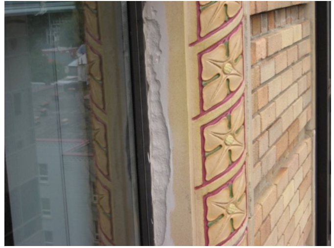
Fig. 3.24: Spalled T.-C. Window Surround
