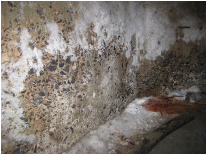
Fig. 3.92: Efflorescence on Foundation Pier
