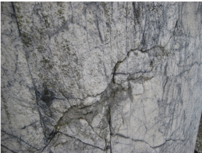
Fig. 2.19: Cracking at Portico Column
