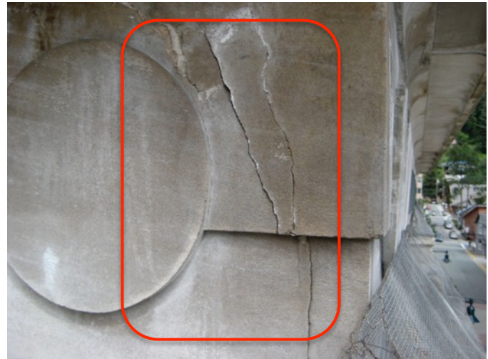
Fig. 1.16: Cracking of Stone Portico Beams
