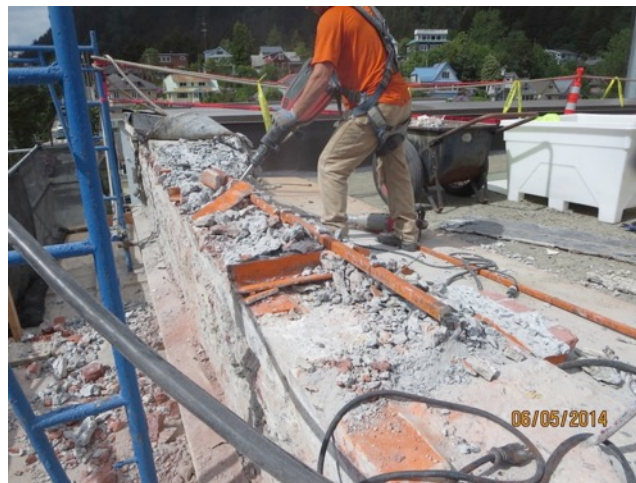
Fig. 5.39: Demolition of Roof Parapet
