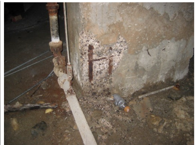
Fig. 3.90: Corrosive Spalling of Pier
