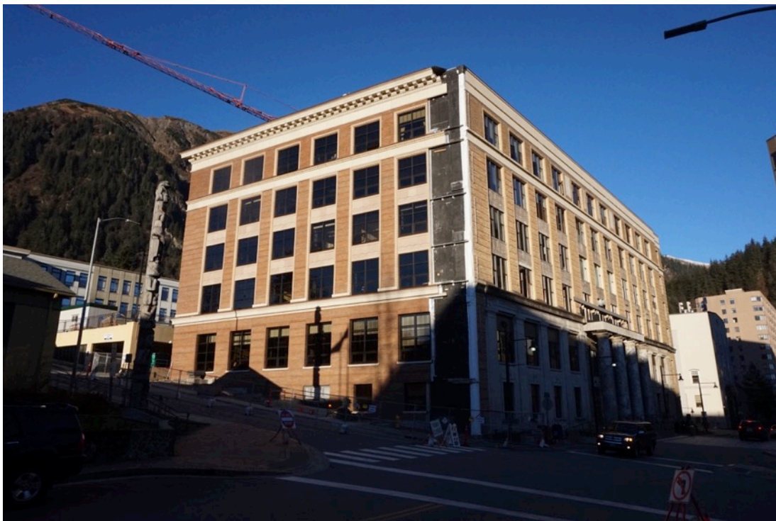
Fig. 6.1: In-Progress Re-Cladding of the Alaska Capitol, West Side New cladding is left of corner, existing building is right of corner.
