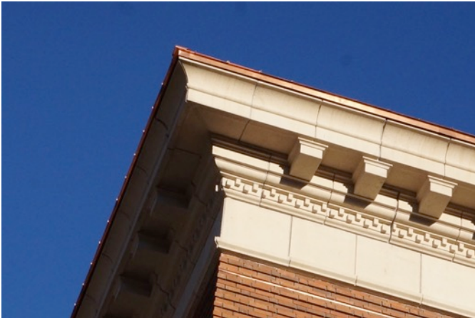
Fig. 6.4: Reconstructed Cornice Band
