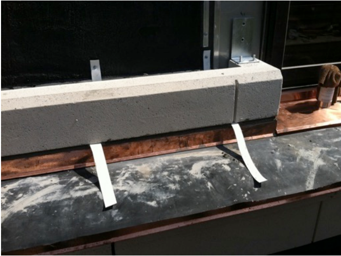
Fig. 5.62: Pre-Cast Conc. Sill With Weeps
