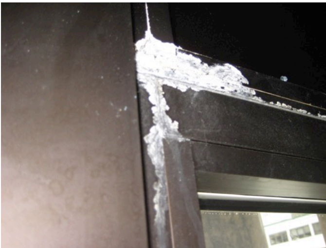
Fig. 3.79: Lime Stains Exuding From Joints
