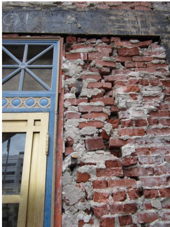
Fig. 5.13: Inner Wythes of Brickwork
