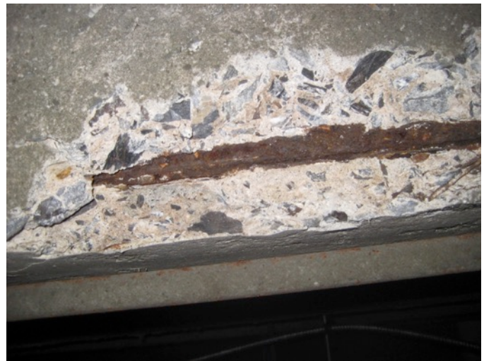
Fig. 3.88: Corrosive Spalling of Fl. Joist
