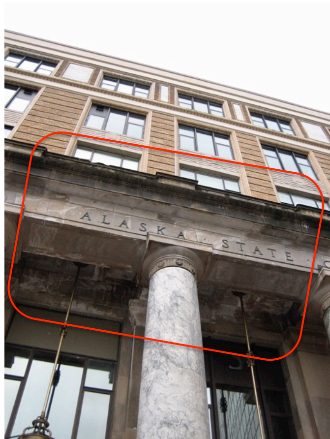
Fig. 2.34: Severe Staining of Portico Ceiling
