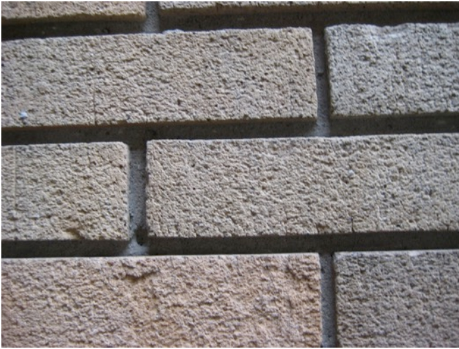
Fig. 3.51: Spalled, Eroded Brick
