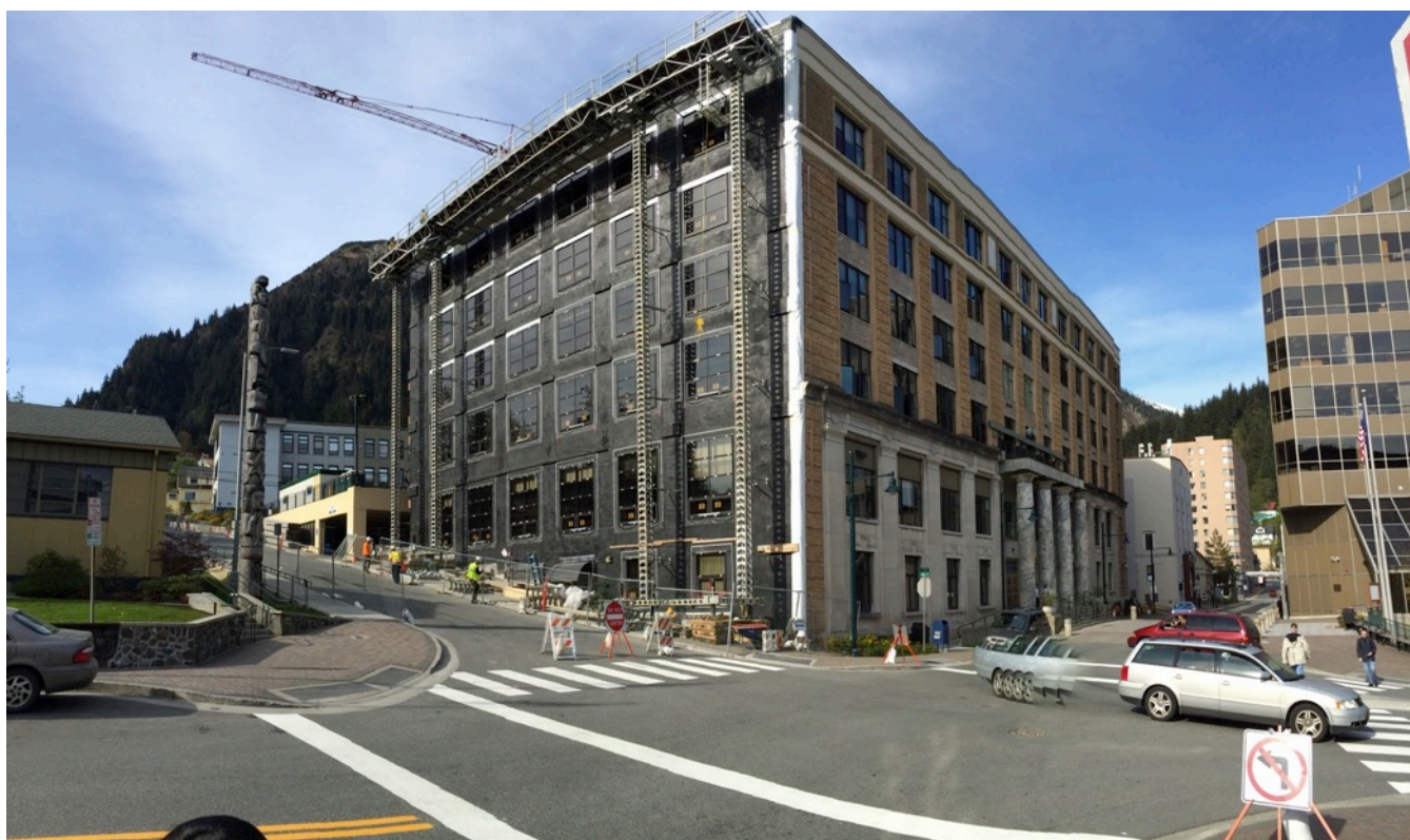
Fig. 5.42: New Concrete Shear Walls & Windows, W. Side
