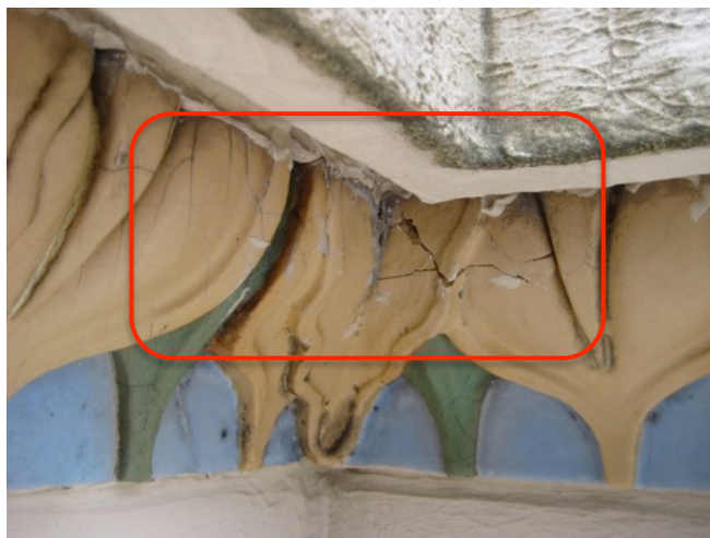
Fig. 3.16: Cracking Level 5 Terra-Cotta Band
