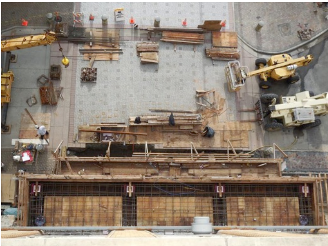
Fig. 5.18: New Portico Formwork & Reinf.
