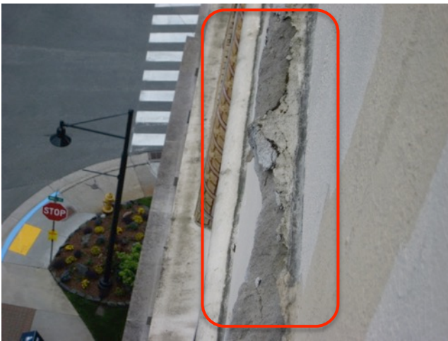
Fig. 3.7: Spalling Roof-Level Band Note sidewalks below.
