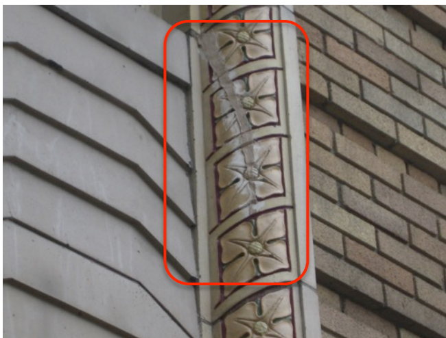
Fig. 3.21: Spalled T.-C. Window Surround
