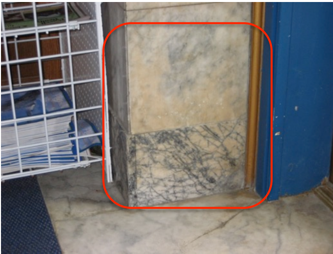
Fig. 2.43: Oxide Stains @ Interior Marble
