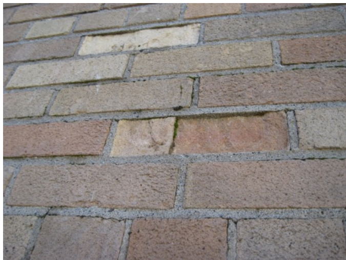
Fig. 3.93: Spalled Brick on 1931 AK. Capitol, Fig. 3.94: Intact Brick on 1904 Seattle Bldg.
