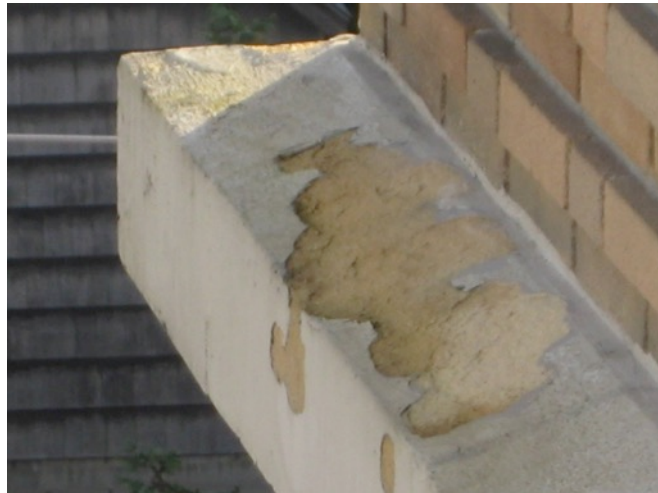
Fig. 3.12: Spalling Level 5 Terra-Cotta Band
