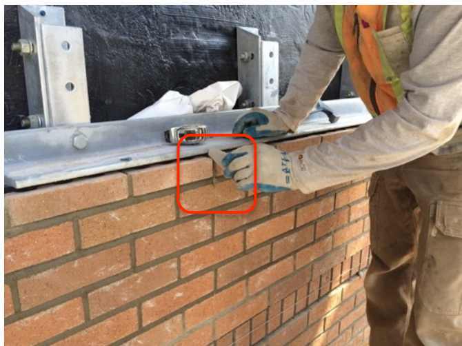
Fig. 5.55: Installing Sloped Panel-Top Vents
