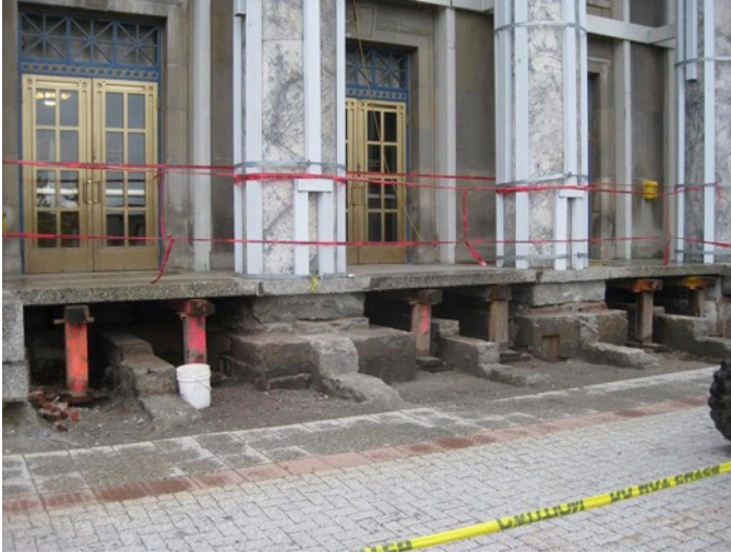
Fig. 5.1: Stairs Removed to Expose Found. Fig. 5.2: Bracing the Marble Columns
