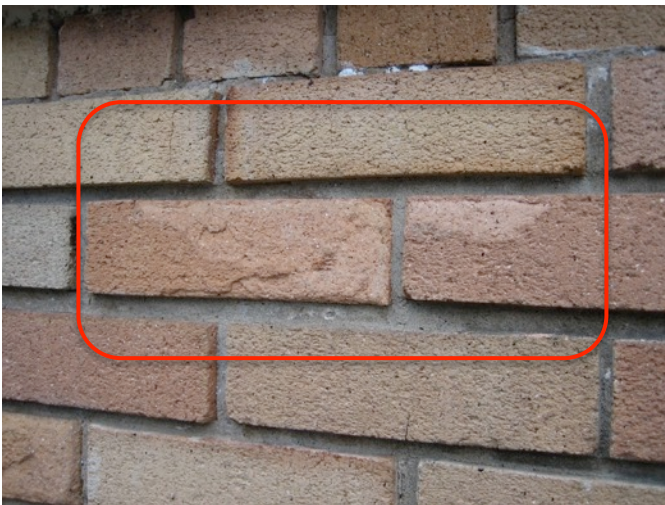
Fig. 1.3: Brick Spalling
