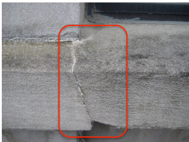
Fig. 3.43: Cracked Stone Sill
