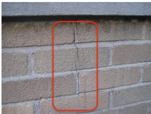
Fig. 3.61: Vertical Brick Cracking
