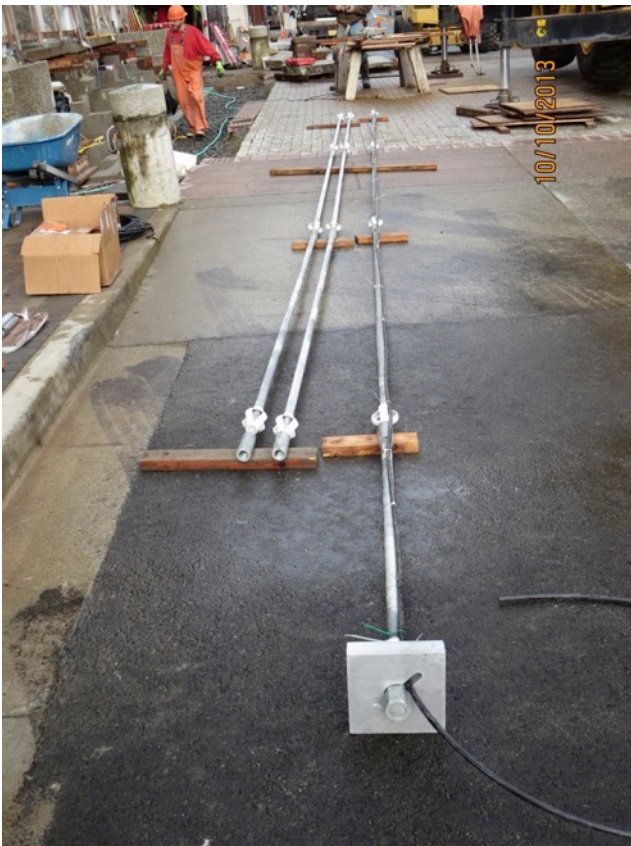
Fig. 5.22: Column Reinforcing Strands
