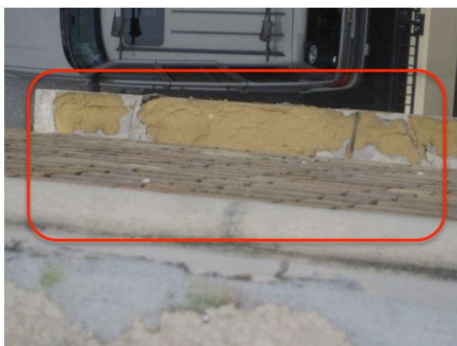
Fig. 3.14: Spalling Level 5 Terra-Cotta Band
