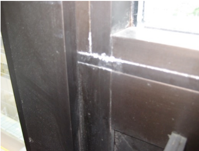
Fig. 3.77: Lime Stains on Window Frame
