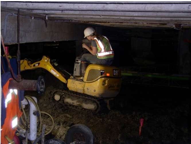
Fig. 5.32: Excavating Crawspace
