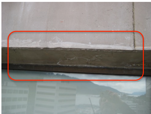
Fig. 3.29: Spalling, Damaged T.-C. Bottom
