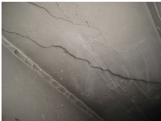
Fig. 3.81: Cracking of Conc. Floor Slab
