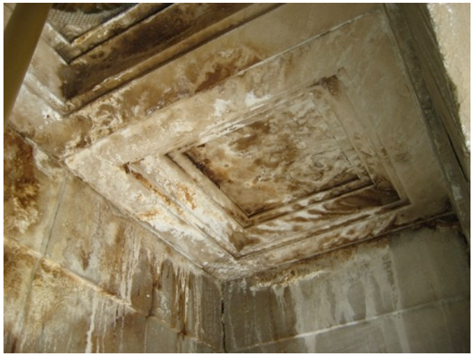
Fig. 2.38: Staining & Erosion of Portico Clg.
