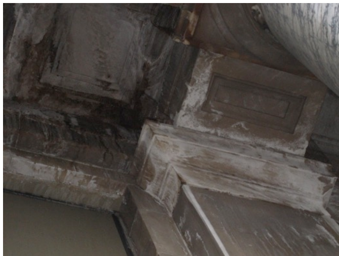
Fig. 2.35: Severe Staining of Portico Ceiling
