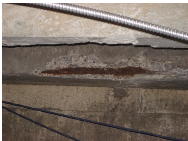
Fig. 3.85: Corrosive Spalling of Fl. Joist
