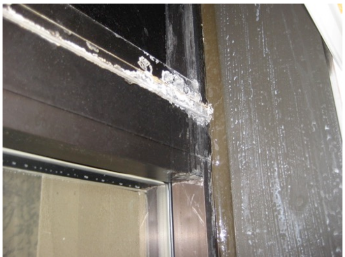
Fig. 2.42: Lime Staining Below Portico Roof
