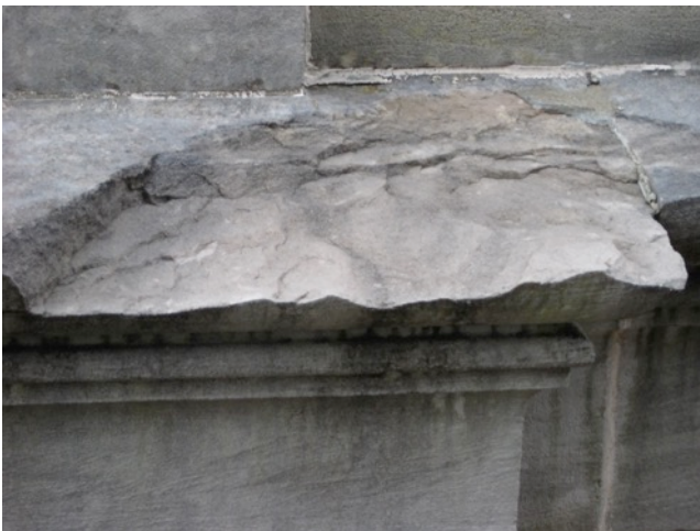
Fig. 3.40: Close-Up of W.-T. Top Delamination
