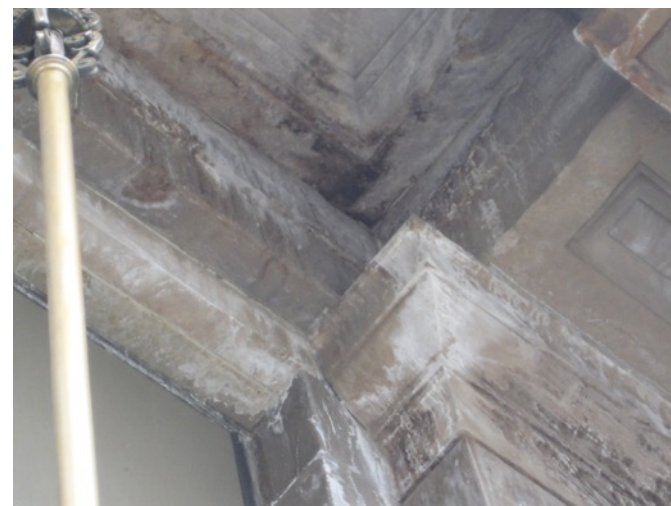
Fig. 2.36: Severe Staining of Portico Ceiling
