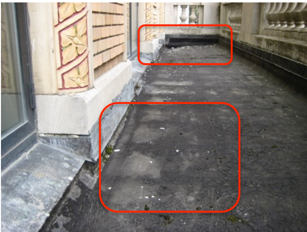
Fig. 3.9: Spalled-Off Pieces on Portico
