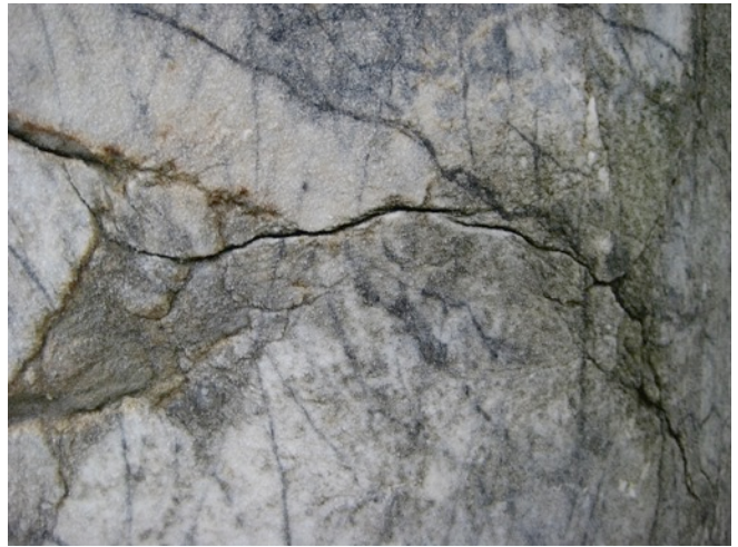
Fig. 2.22: Cracking at Portico Column
