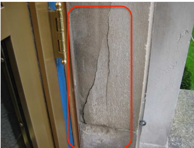
Fig. 2.9: Cracked Middle of Struct. Pilstr.
