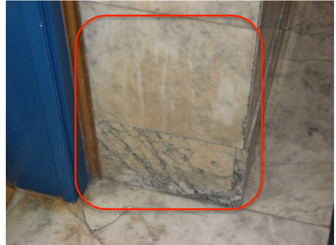
Fig. 2.44: Oxide Stains @ Interior Marble
