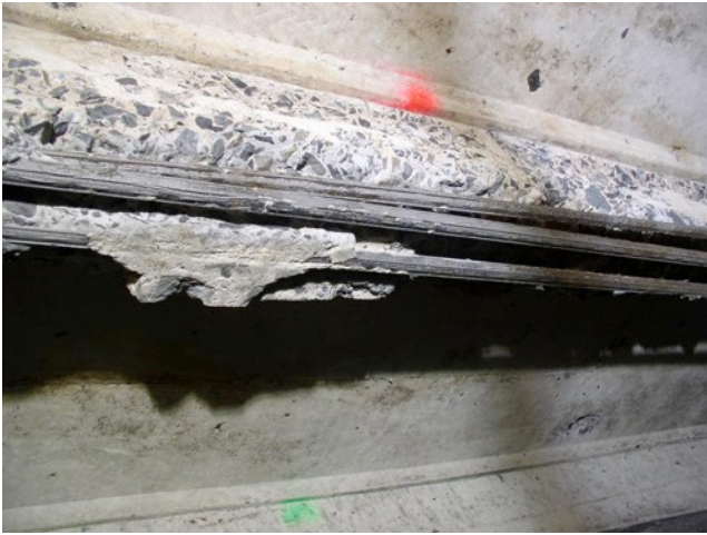
Fig. 5.34: Cleaned-Off Joist Reinforcing
