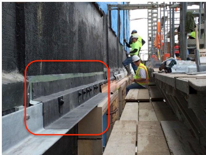
Fig. 5.53: EPDM Membrane Over Ledgers
