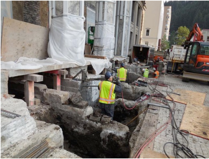
Fig. 5.14: Drilling of Portico Foundations
