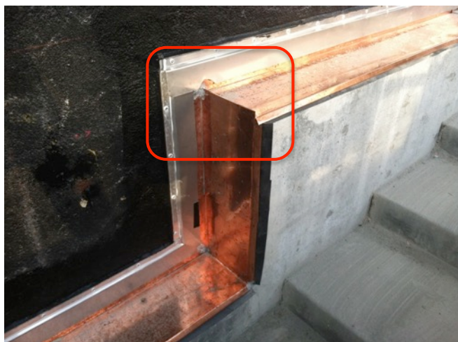
Fig. 5.45: New Thr.-Wall Copper Flsh'gs.
