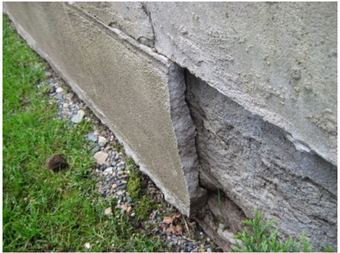
Fig. 1.2: Degradation of Stone Base
