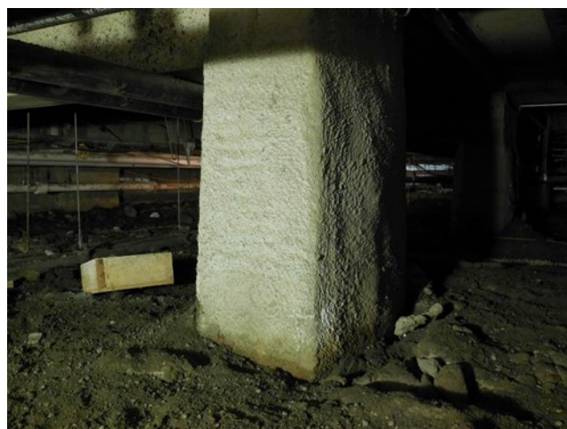
Fig. 5.37: Repaired Concrete Pier
