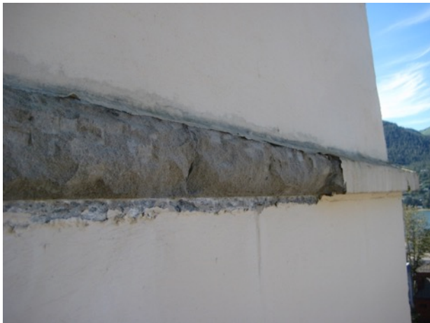
Fig. 3.4: Spalling Roof-Level Band
