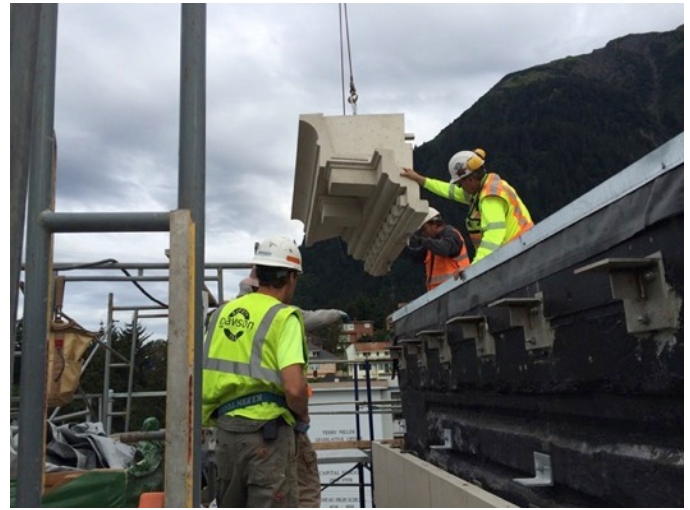
Fig. 5.77: Placing Upper Cornice Band
