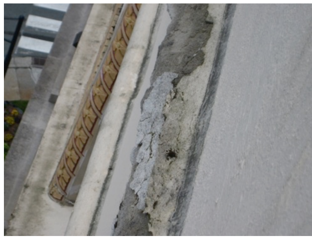
Fig. 3.8: Spalling Roof-Level Band Note sidewalks below.
