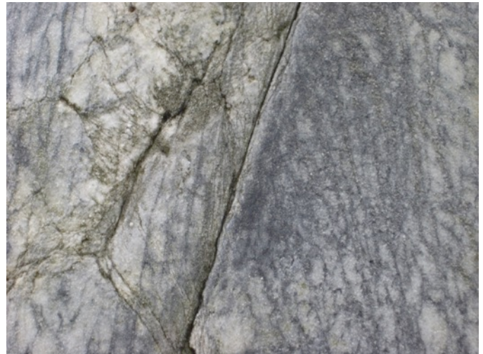
Fig. 2.20: Cracking at Portico Column
