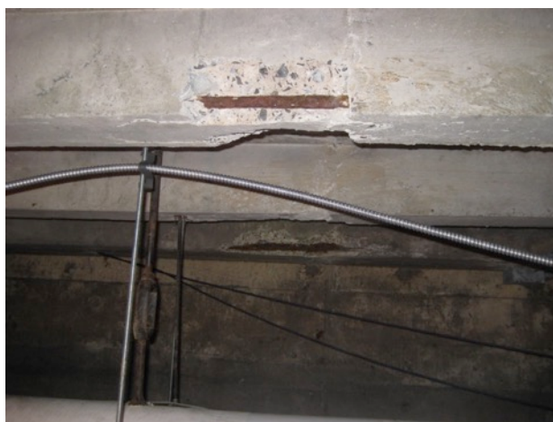
Fig. 3.84: Corrosive Spalling of Fl. Joist
