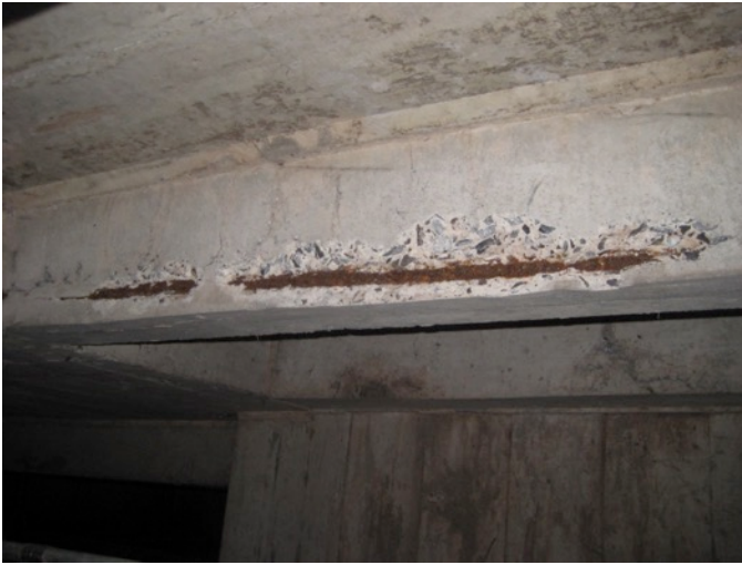
Fig. 3.87: Corrosive Spalling of Fl. Joist
