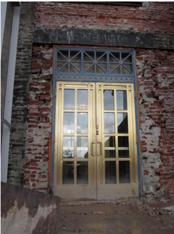
Fig. 5.12: Inner Wythes of Brickwork
