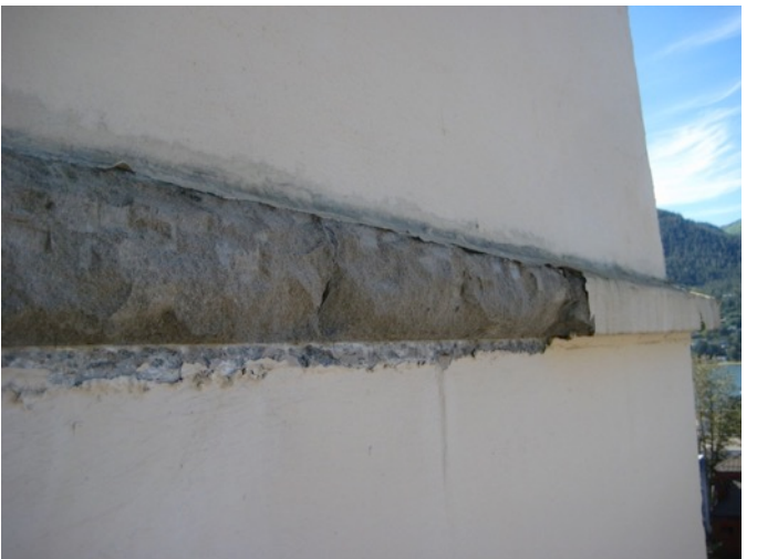
Fig. 1.10: Spalling Stone Cornice Band
