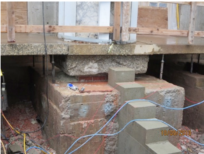
Fig. 5.16: New Portico Stair Foundations
