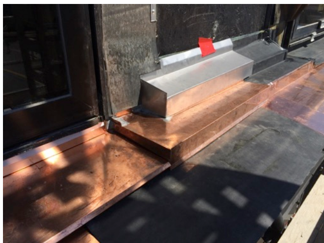
Fig. 5.61: Water-Table Flashings
