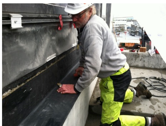
Fig. 5.44: EPDM Membrane Caps Ledges
