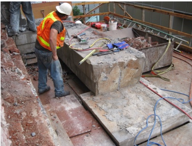
Fig. 5.7: Demolition of Portico Beam
