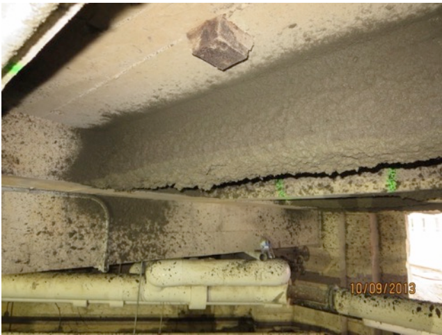
Fig. 5.36: Repaired Floor Joist
