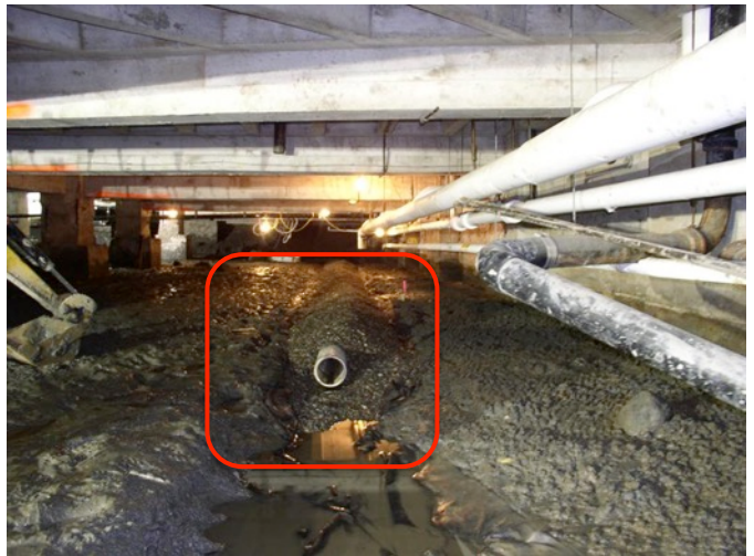
Fig. 5.33: Crawspace Drainage System
