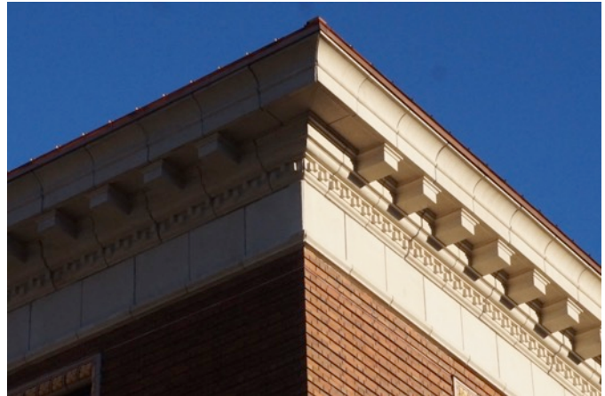
Fig. 6.5: Reconstructed Cornice Band
