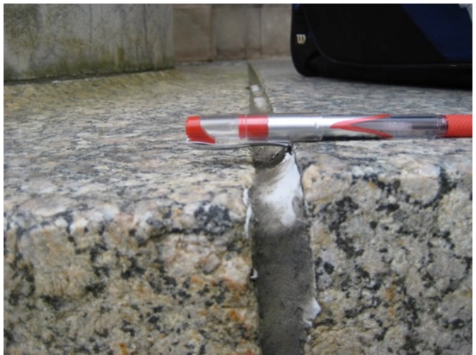
Fig. 2.24: Downward Displacement Bel. Col.
