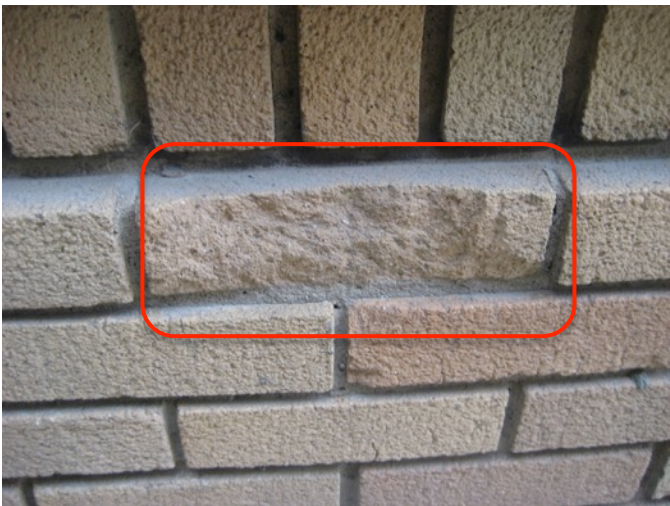
Fig. 3.53: Spalled, Eroded Brick
