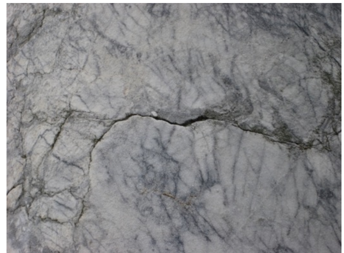
Fig. 2.18: Cracking at Portico Column
