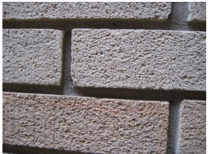
Fig. 1.8: Brick Surface Erosion
