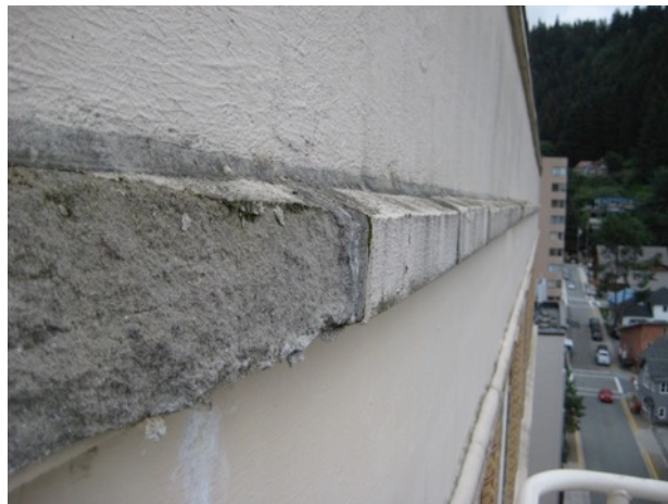
Fig. 3.2: Spalling Roof-Level Band
