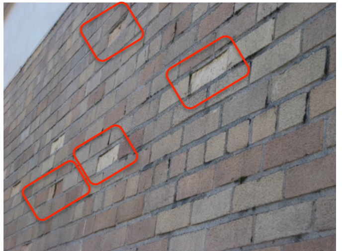
Fig. 3.54: Spalled Brick
