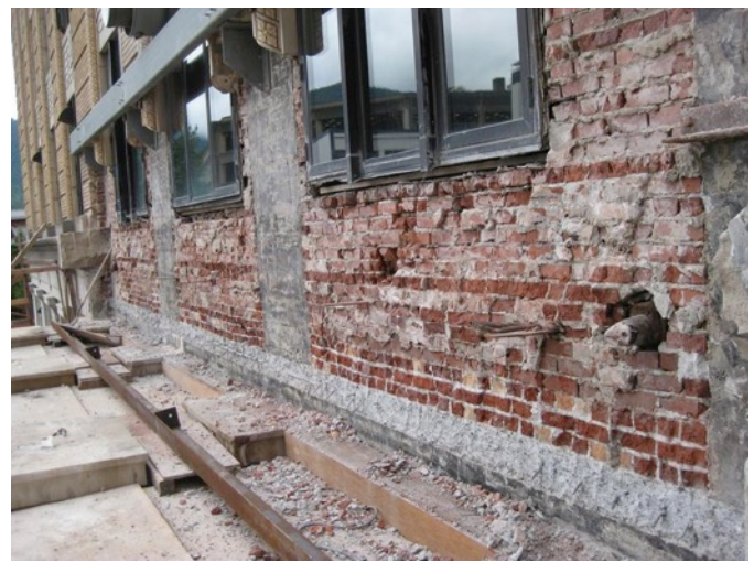
Fig. 5.6: Demolition of Building Masonry
