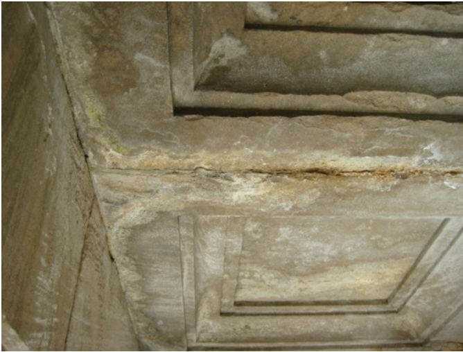
Fig. 2.37: Staining & Erosion of Portico Clg.
