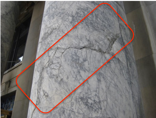
Fig. 2.17: Cracking at Portico Column
