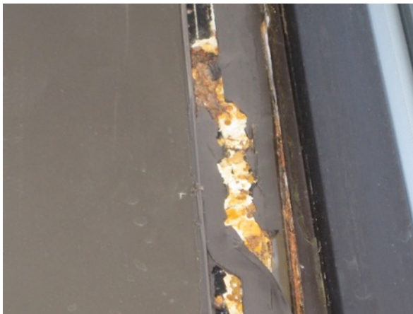
Fig. 3.70: Steel Jamb Corrosion
