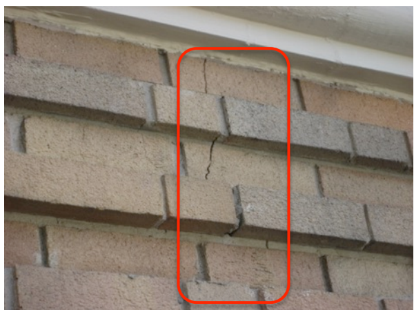
Fig. 3.59: Vertical Brick Cracking
