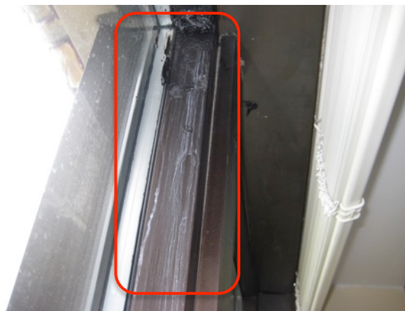
Fig. 3.71: Lime Stains on Mullion
