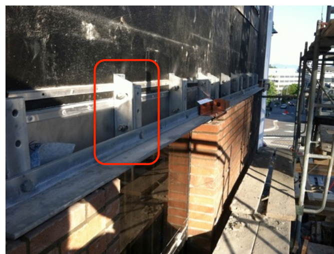
Fig. 5.52: Adjust. Dbl.-Angle Ledger Furring
