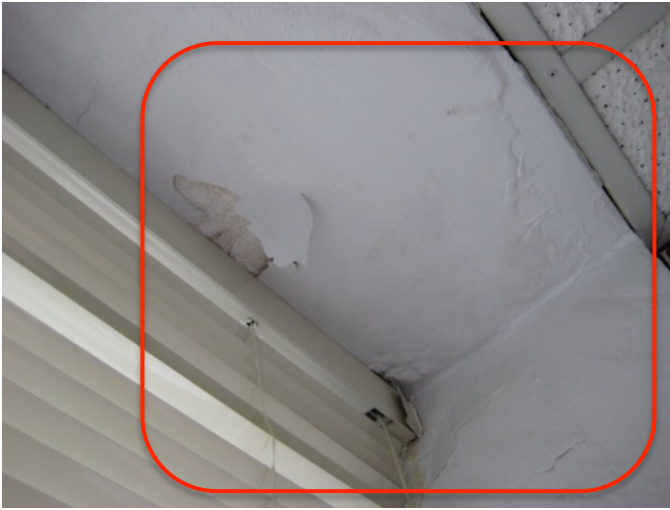
Fig. 3.75: Plaster Damage Above Wind. Head
