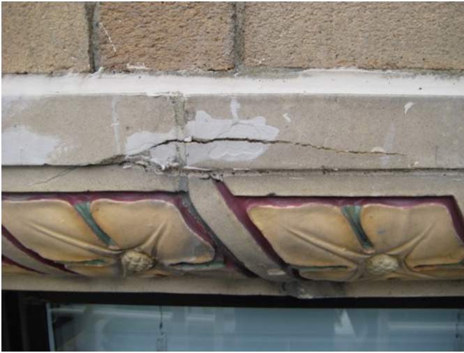
Fig. 3.23: Spalled T.-C. Window Surround
