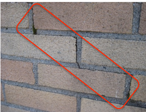
Fig. 3.62: Stair-Step Cracking
