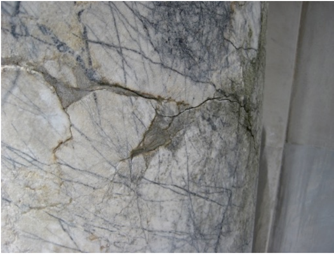
Fig. 2.21: Cracking at Portico Column
