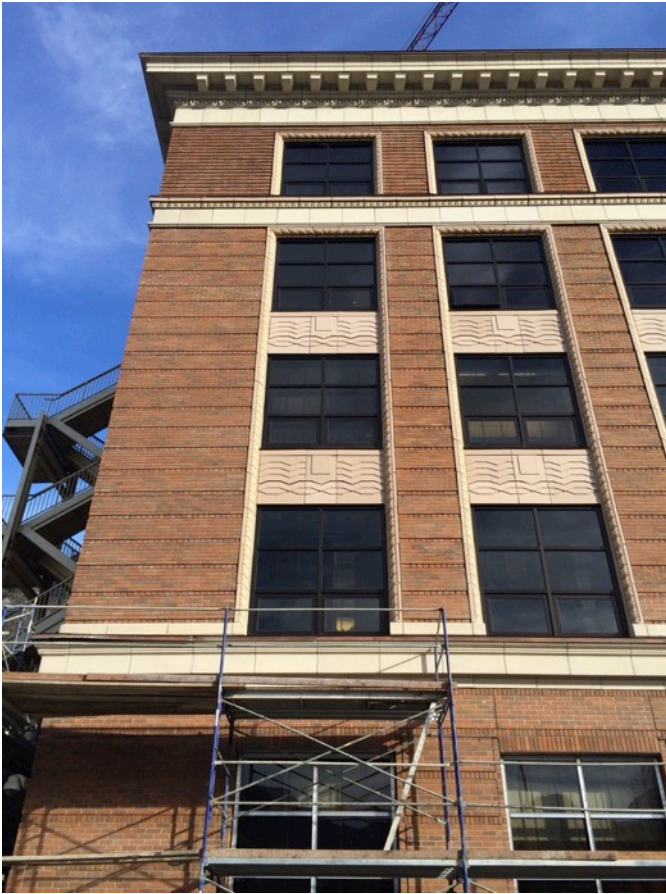
Fig. 6.2: New Cladding on West Side
