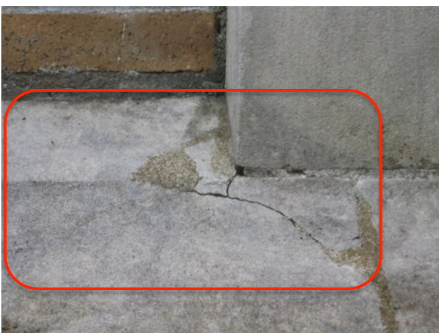
Fig. 3.38: Water-Table Top Delamination
