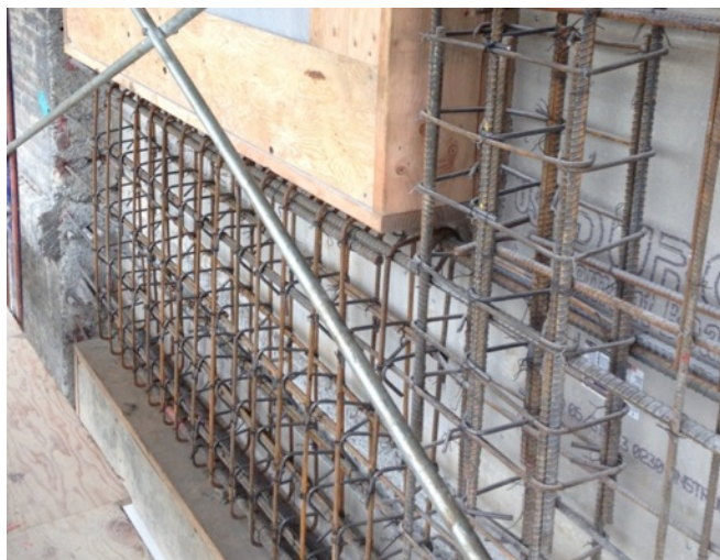
Fig. 5.40: New Shear Wall Reinforcing
