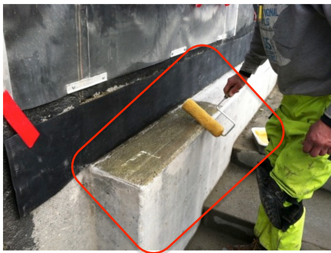
Fig. 5.43: New Concrete Support Ledge
