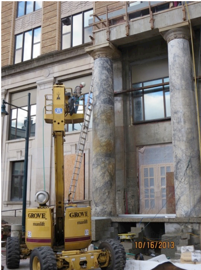
Fig. 5.24: Grouting Column Reinforcing
