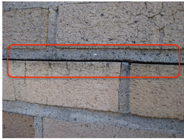
Fig. 3.64: Horiz. Crack @ Sagging Lintel
