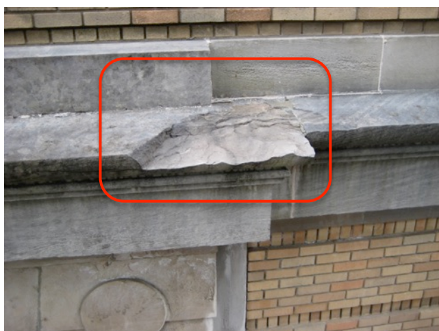
Fig. 3.39: Water-Table Top Delamination
