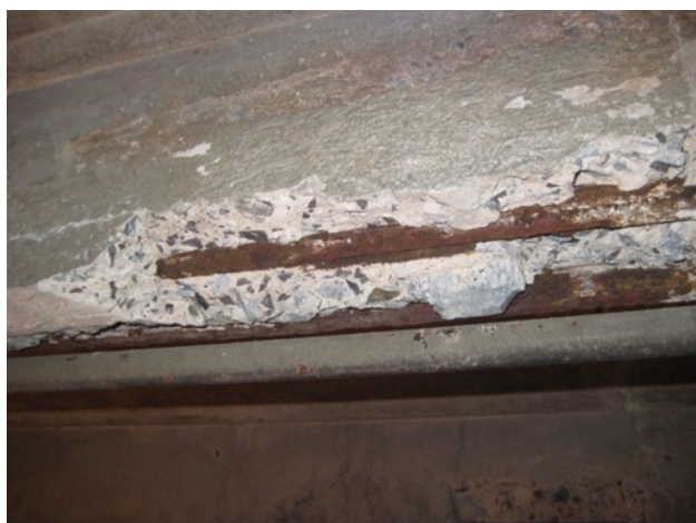
Fig. 3.83: Corrosive Spalling of Fl. Joist
