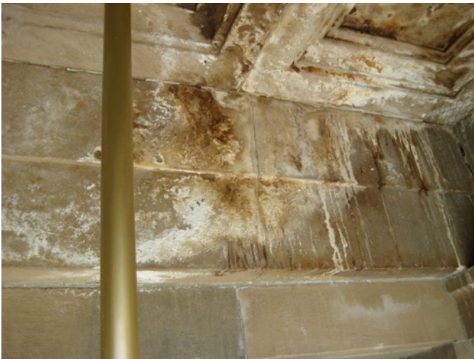
Fig. 2.39: Staining & Erosion of Portico Clg.
