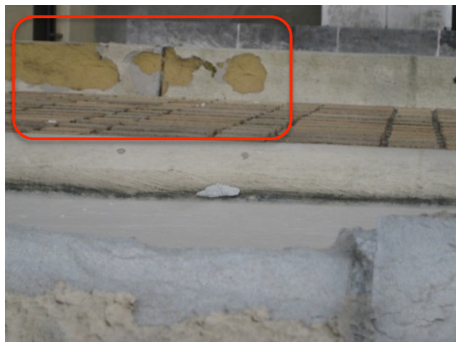
Fig. 3.15: Spalling Level 5 Terra-Cotta Band
