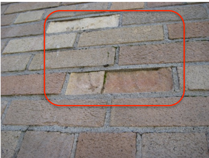
Fig. 3.55: Spalled, Eroded Brick
