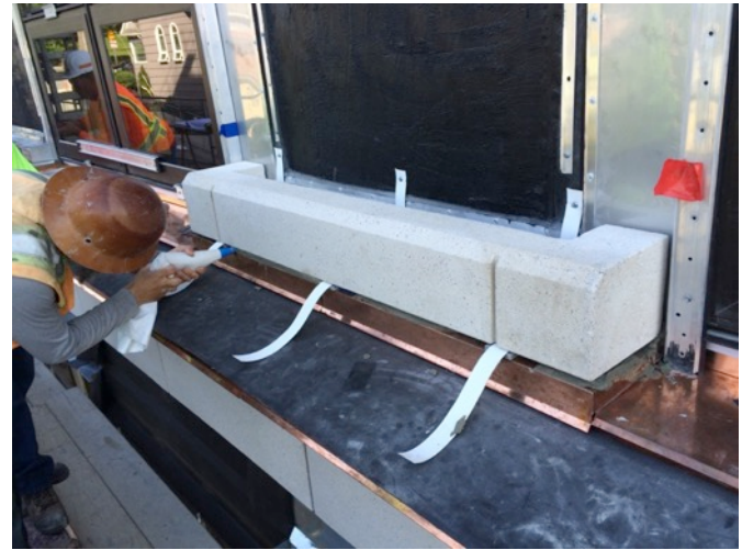
Fig. 5.63: Pre-Cast Conc. Sill With Weeps
