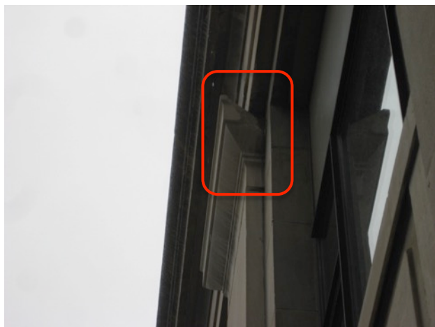
Fig. 3.41: Spalled Pilaster Capital
