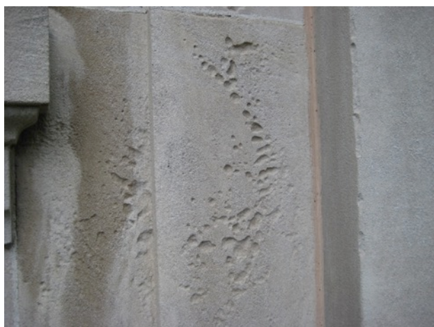
Fig. 3.45: Differential Surface Erosion
