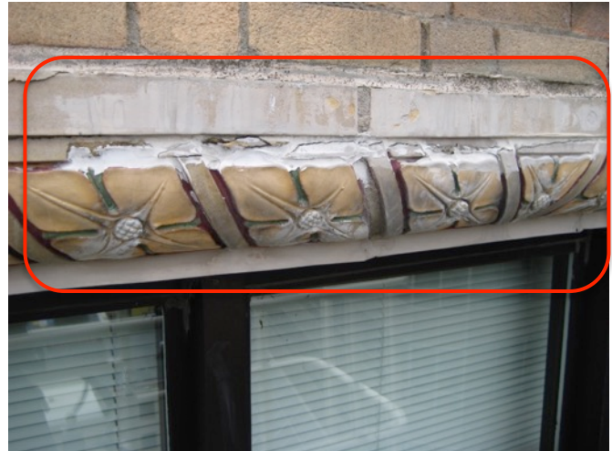
Fig. 3.22: Spalled T.-C. Window Surround
