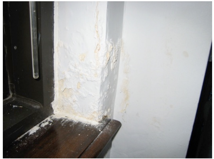
Fig. 1.12: Water Infiltration to Interior
