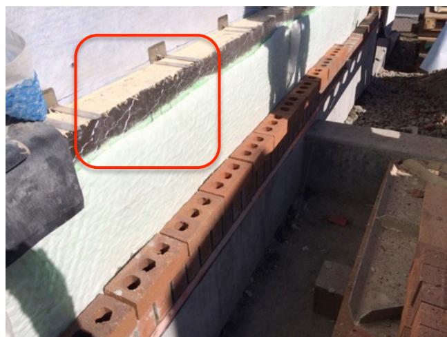
Fig. 5.48: Insul. & Drain. Mat Layers @ Brick
