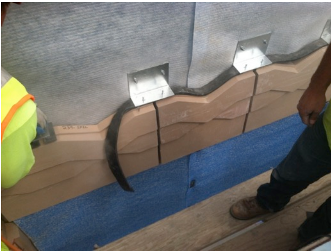
Fig. 5.68: Start of T.-C. Spandrel Installation Fig. 5.69: Terra-Cotta Spandrel Installation
