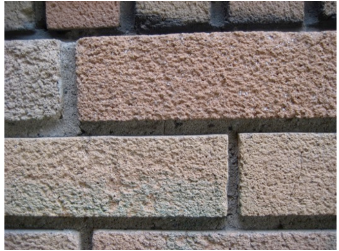
Fig. 3.52: Eroded Brick
