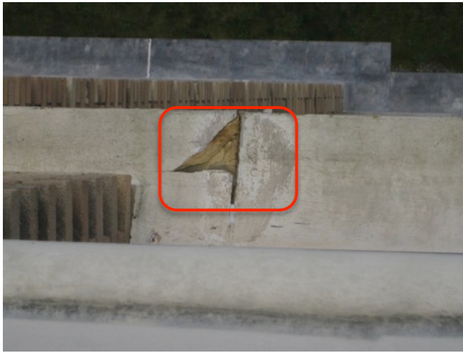
Fig. 3.17: Spalling Level 5 Terra-Cotta Band
