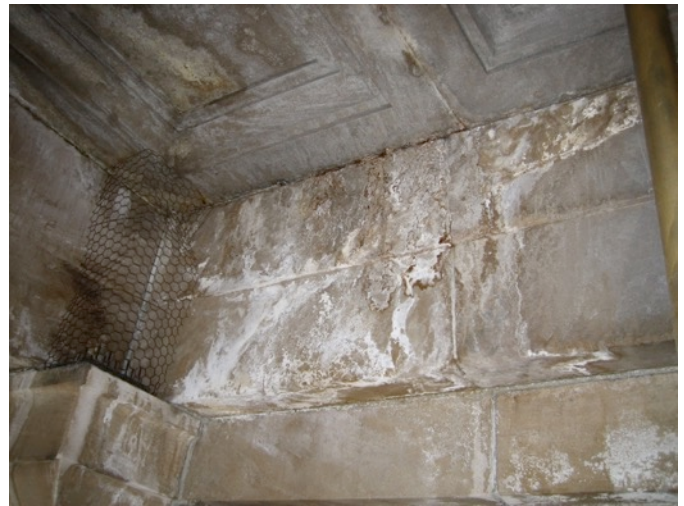
Fig. 1.14: Water Infiltration Into Portico Clg.
