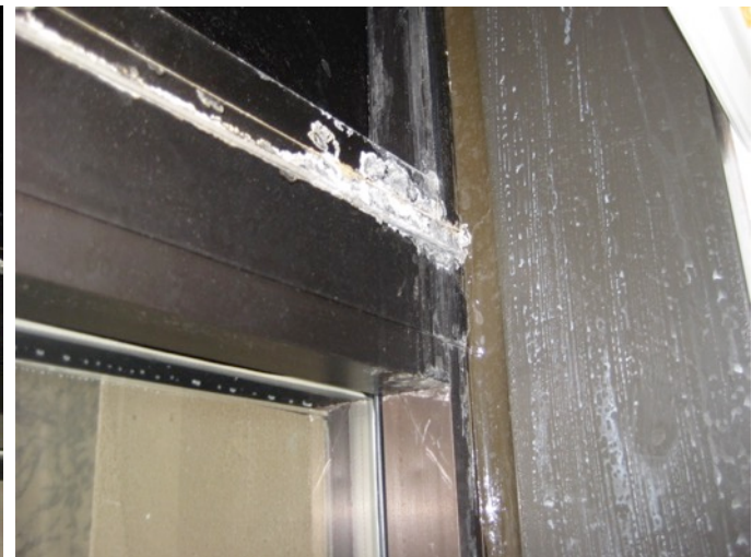
Fig. 3.80: Lime Stains on Window Frame
