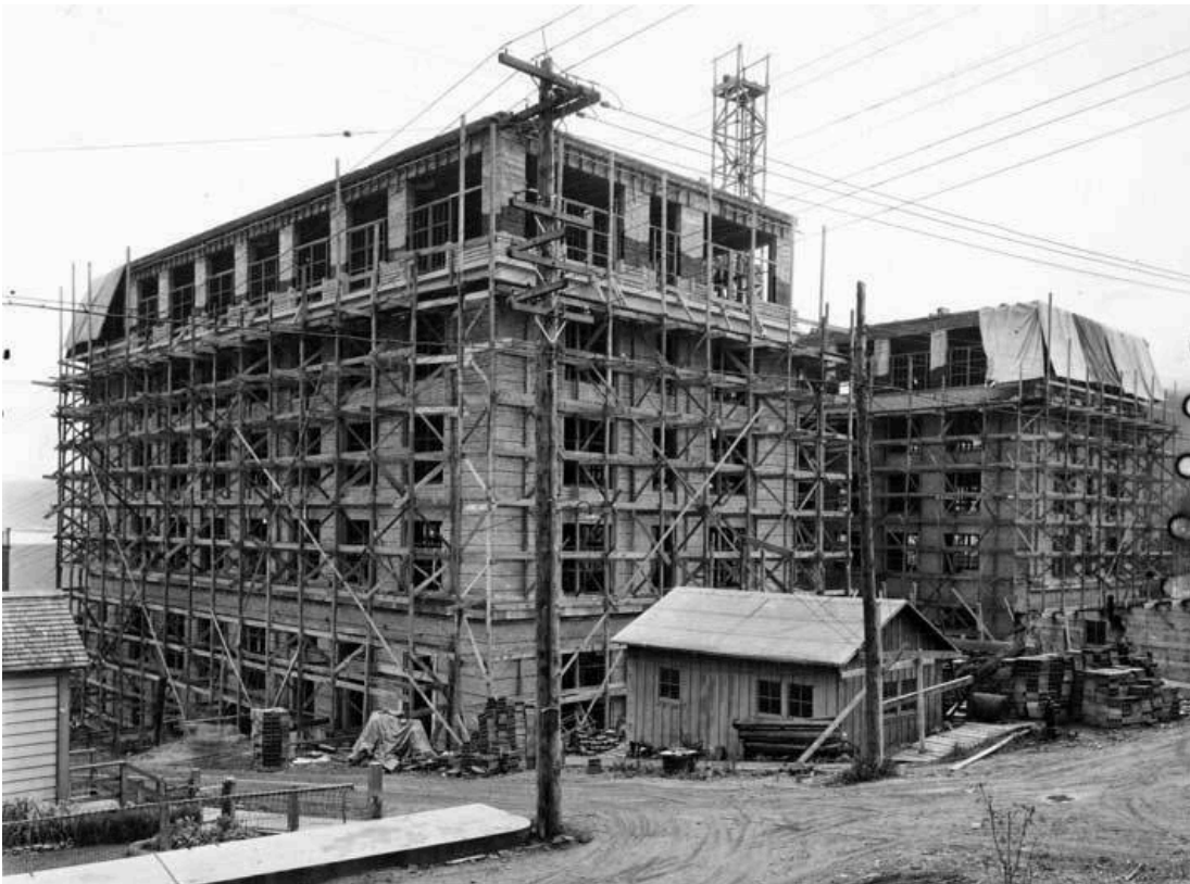
Fig. 0.4: Masonry Exterior Walls Under Construction, Using Wood Scaffolding, 1930
