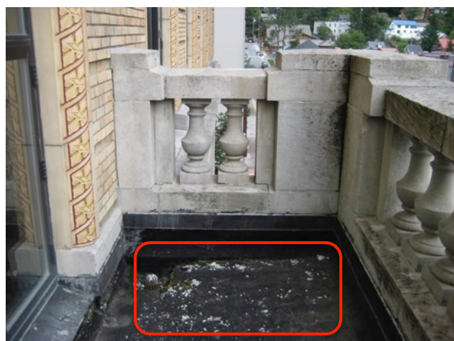
Fig. 3.10: Spalled-Off Pieces on Portico Roof
