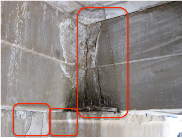
Fig. 2.5: Cracked Stone Beam & Header
