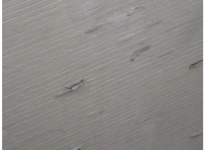
Fig. 3.56: Spalled, Painted Brick Note that brick was coated to limit leakage.
