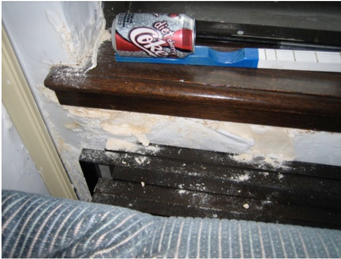
Fig. 1.11: Water Infiltration to Interior
