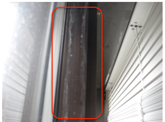
Fig. 3.78: Lime Stains on Mullion
