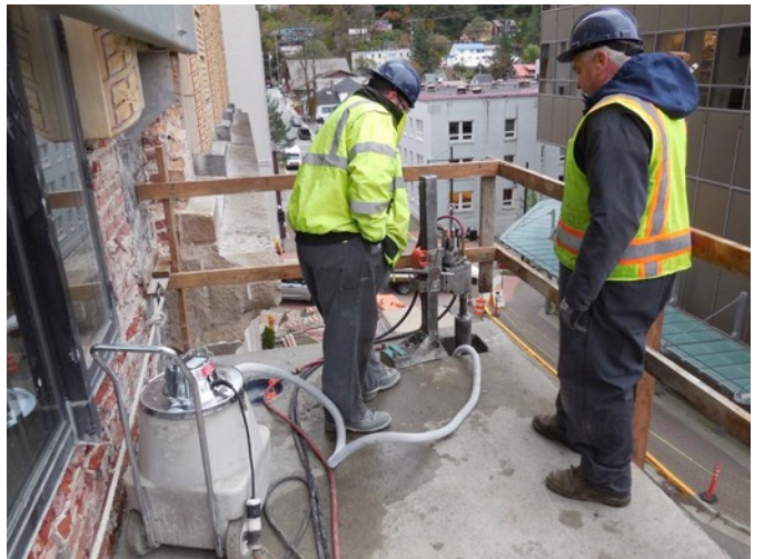
Fig. 5.19: Core-Drilling Marble Columns
