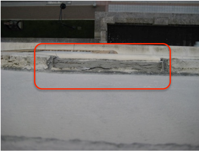
Fig. 3.5: Spalling Roof-Level Band Note “ready-to-fall” piece.
