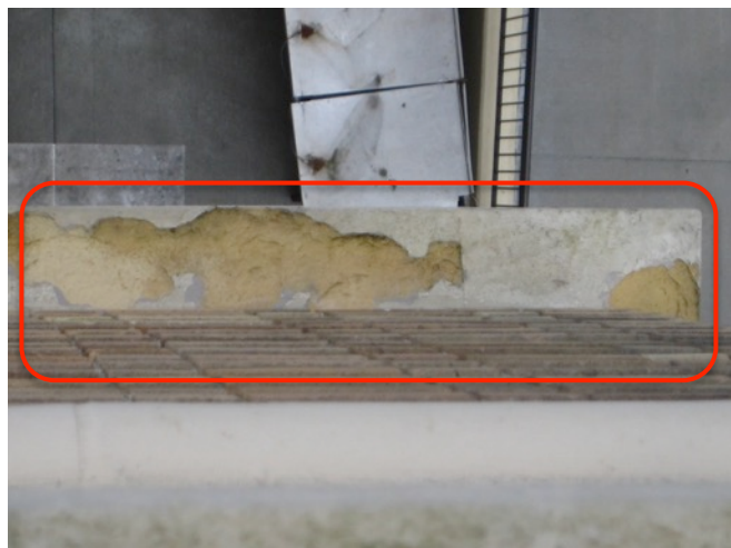
Fig. 3.13: Spalling Level 5 Terra-Cotta Band
