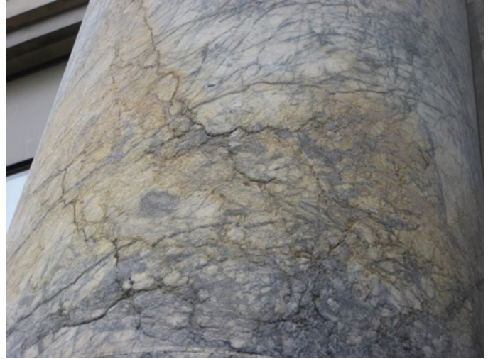
Fig. 2.16: Staining, Cracking at Portico Col.
