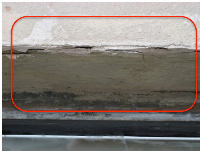
Fig. 3.30: Spalling, Damaged T.-C. Bottom
