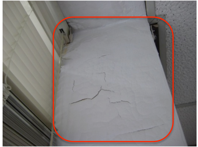
Fig. 3.76: Plaster Damage on Jamb
