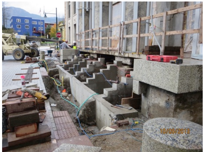
Fig. 5.17: New Portico Stair Foundations
