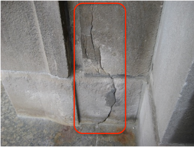
Fig. 2.11: Cracked Base of Struct. Pilaster
