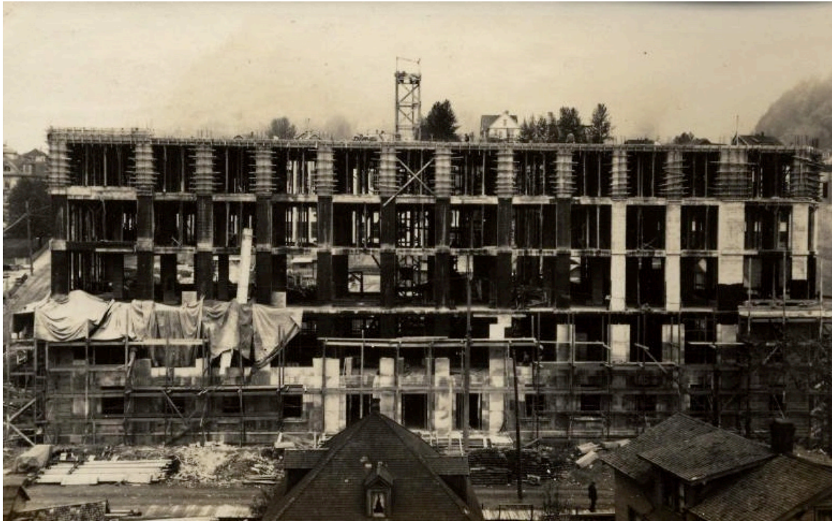
Fig. 0.2: Concrete Skeleton Under Construction, 1930
