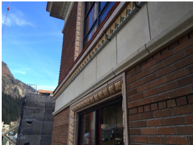
Fig. 5.72: Level 5 Water-Table Band
