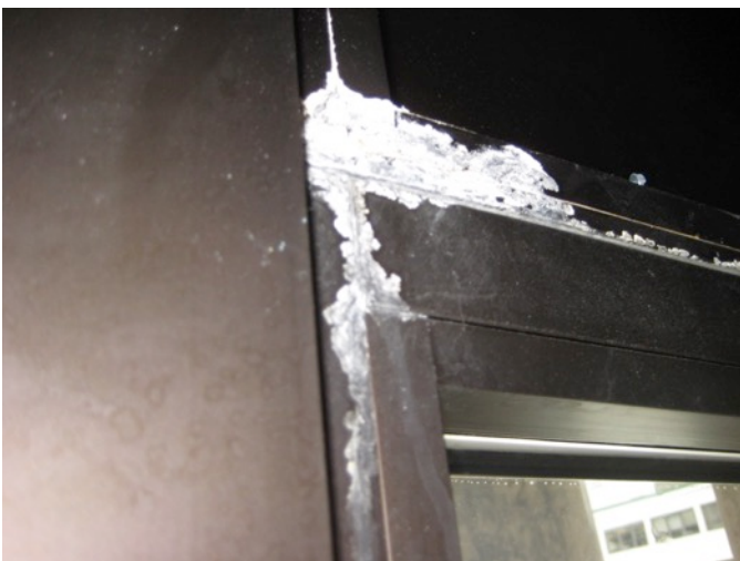
Fig. 2.41: Lime Stains @ Window Bel. Port.
