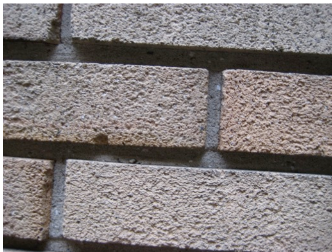
Fig. 3.50: Eroded Brick
