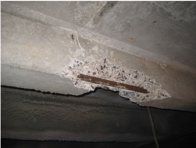
Fig. 3.89: Corrosive Spalling of Fl. Joist
