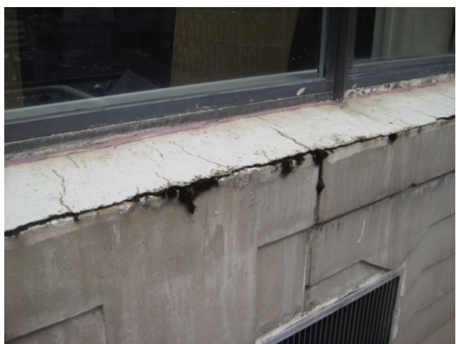
Fig. 3.33: Failing Cement-Wash Sill
