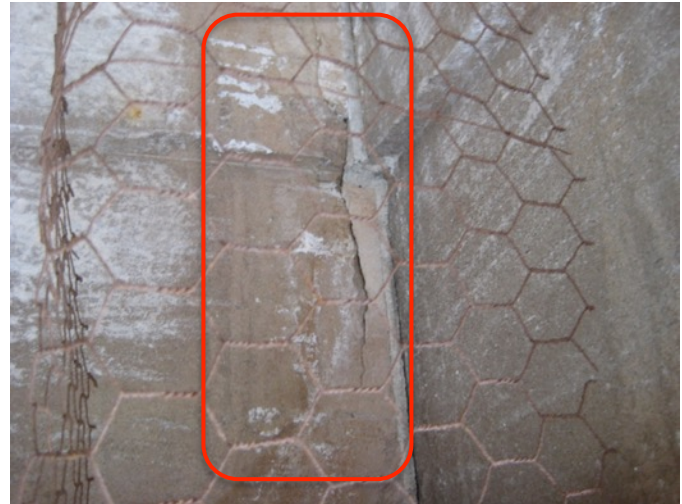
Fig. 2.4: Cracking of Stone Portico Beams
