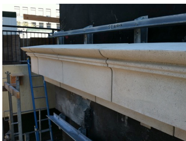
Fig. 5.58: Level 2 Water-Table In-Progress
