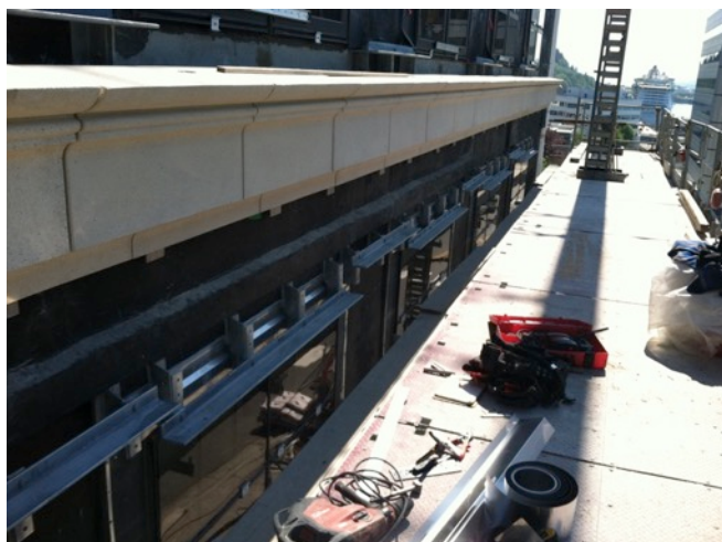
Fig. 5.57: Level 2 Water-Table In-Progress
