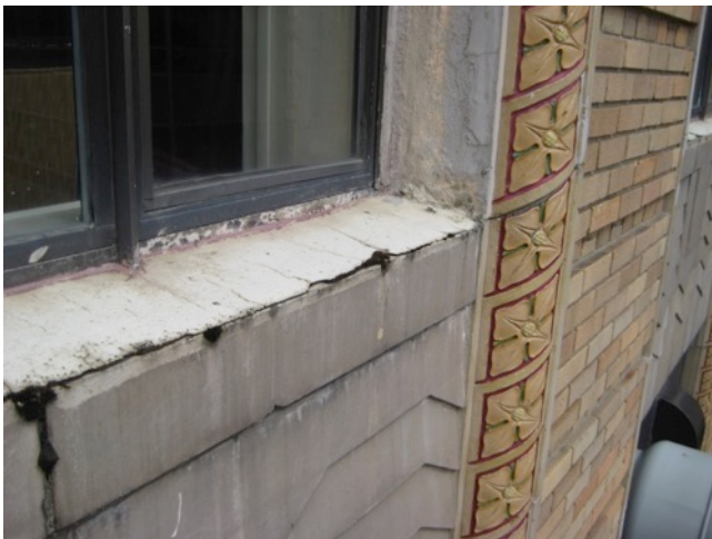
Fig. 3.34: Failing Cement-Wash Sill
