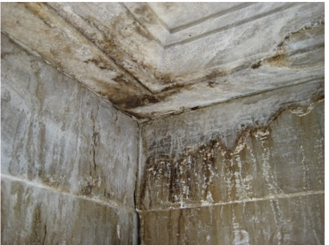
Fig. 2.40: Staining & Erosion of Portico Clg.
