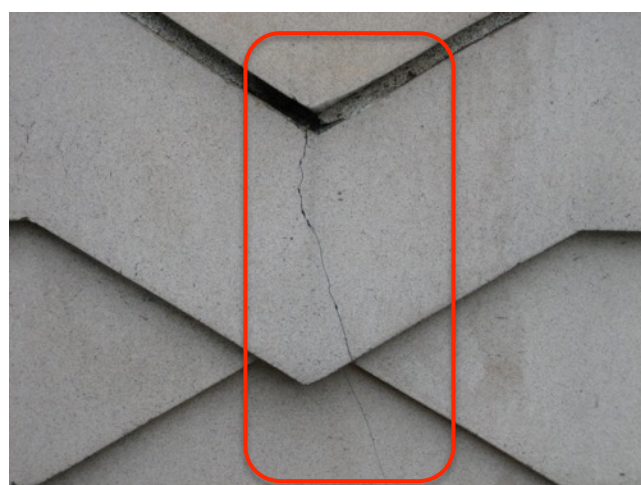
Fig. 3.32: Cracked T.-C. Spandrel Panel
