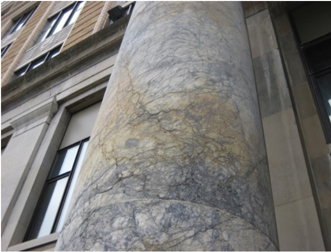
Fig. 2.15: Staining, Cracking at Portico Col.
