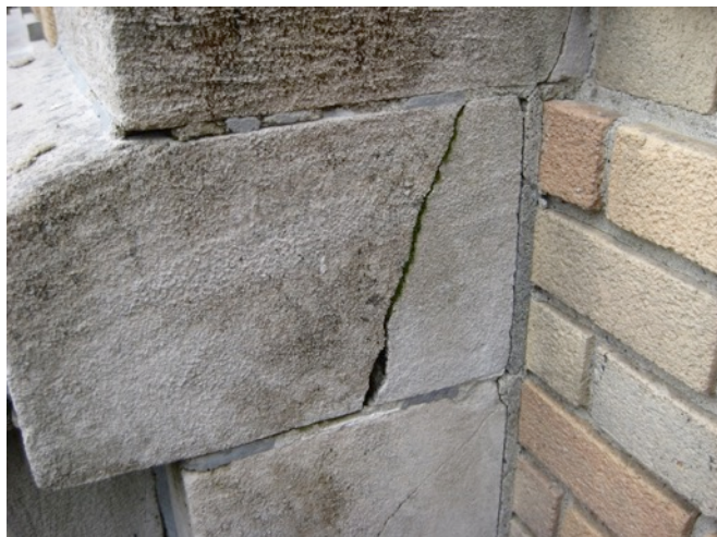
Fig. 2.30: Cracking at Portico Railing
