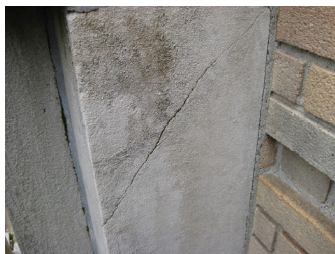
Fig. 2.32: Cracking at Portico Railing
