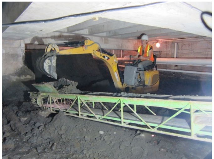
Fig. 5.31: Excavating Crawspace
