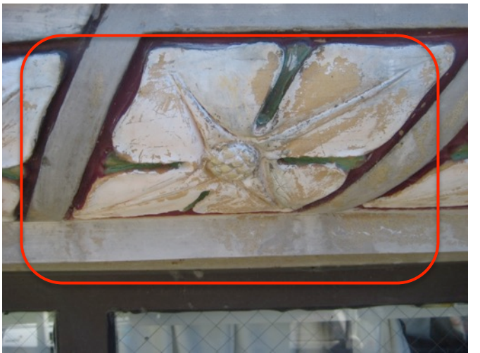
Fig. 3.28: Lime-Stained Window Surround
