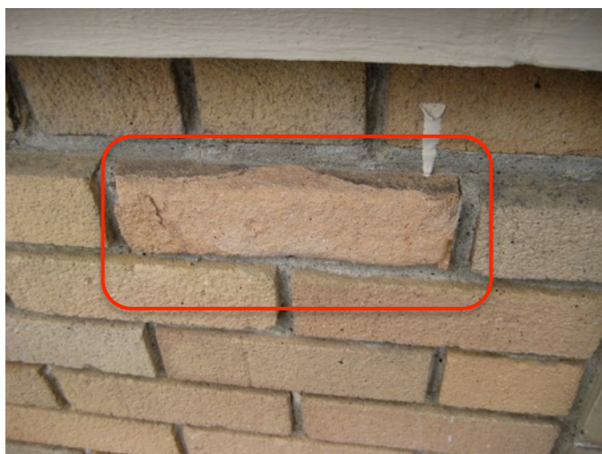
Fig. 3.47: Spalled, Eroded Brick
