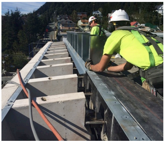
Fig. 5.79: Installed Upper Cornice Band
