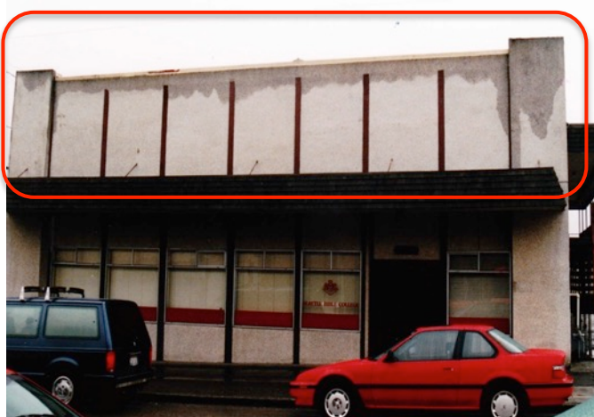
Fig. 3.99 Wetting Pattern on Lee Side
