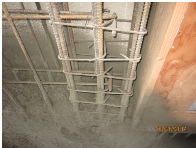
Fig. 5.41: Shot-Creting New Shear Walls
