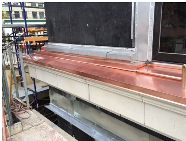
Fig. 5.62: Water-Table Flashings
