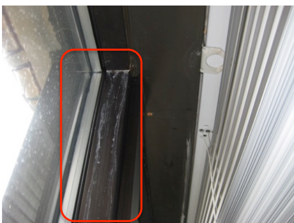
Fig. 3.72: Lime Stains on Mullion
