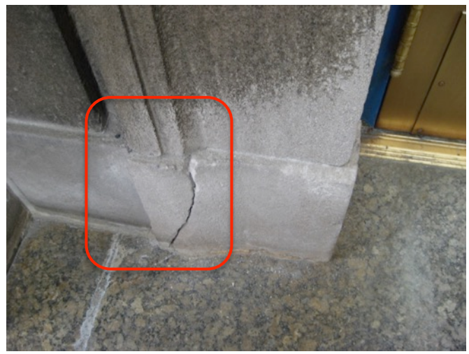
Fig. 2.12: Cracked Base of Struct. Pilaster
