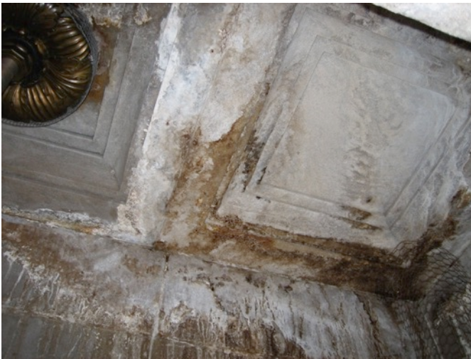
Fig. 1.13: Water Infiltration Into Portico Clg.
