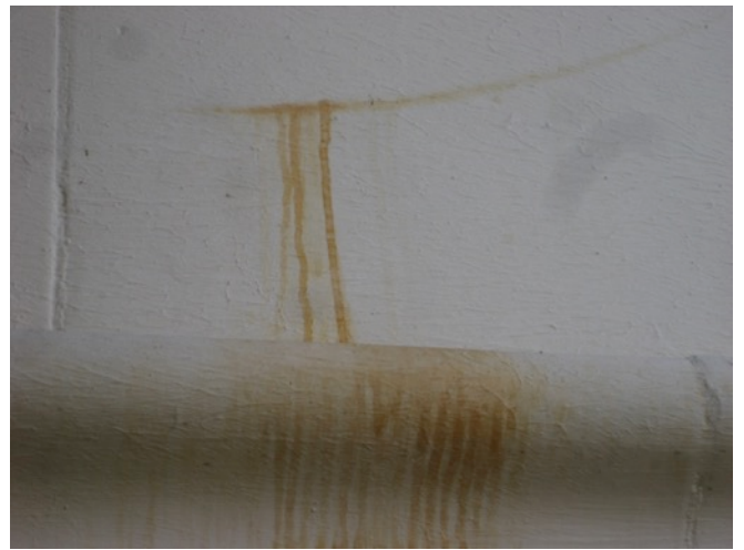
Fig. 3.20: Close-Up of Oxide Stain @ T.-C.
