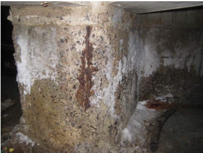
Fig. 3.91: Corrosive Spalling, Efflor. of Pier
