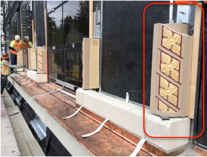
Fig. 5.66: Start of T.-C. Window Surr. Install. Fig. 5.67: Terra-Cotta Window Head
