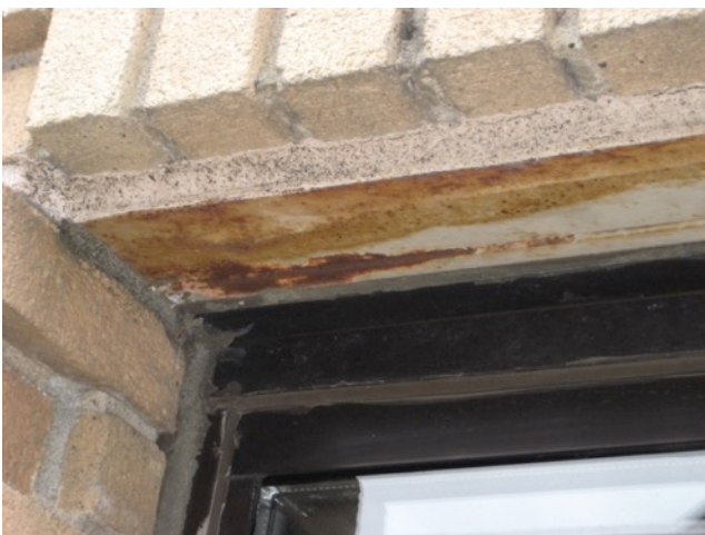
Fig. 3.67: Lintel Corrosion
