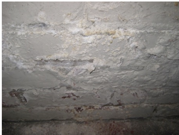
Fig. 3.57: Spalling & Efflor. on Int. Face Fig. 3.58: Spalling & Efflor. on Interior Face
